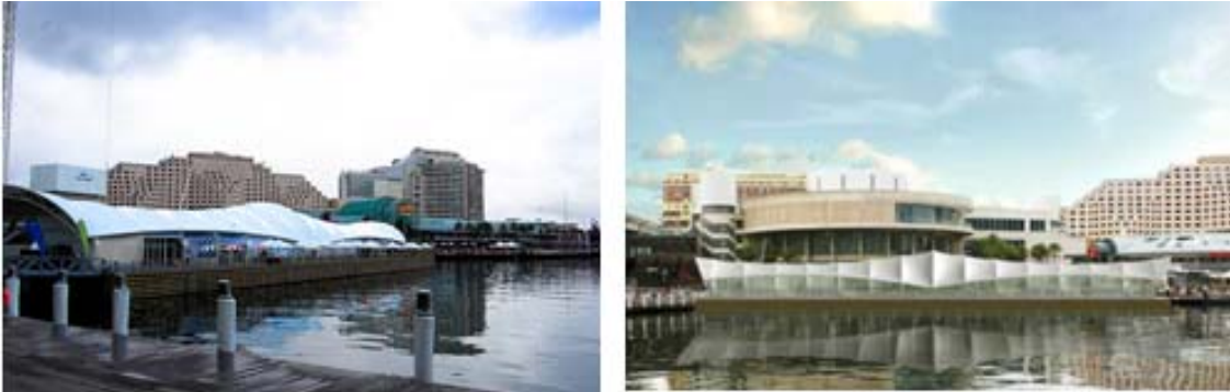
Figure 11: Existing Structures – Dockside Pavilion
