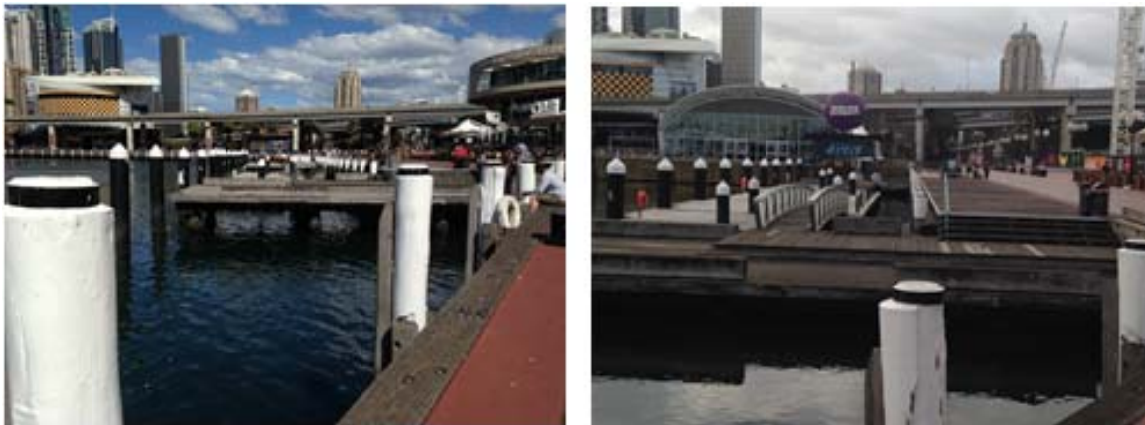
Figure 9: Existing Structures – Convention Wharf
