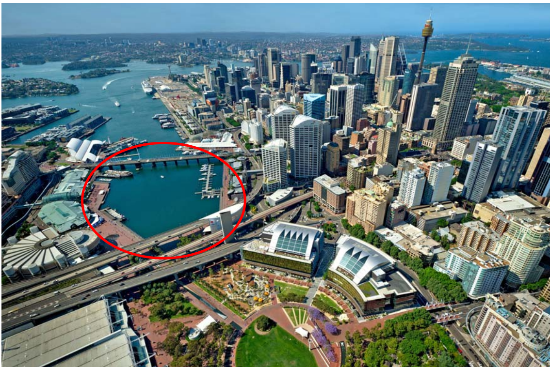
Figure 1: Aerial Photo showing Location of Cockle Bay relative to Sydney's CBD
