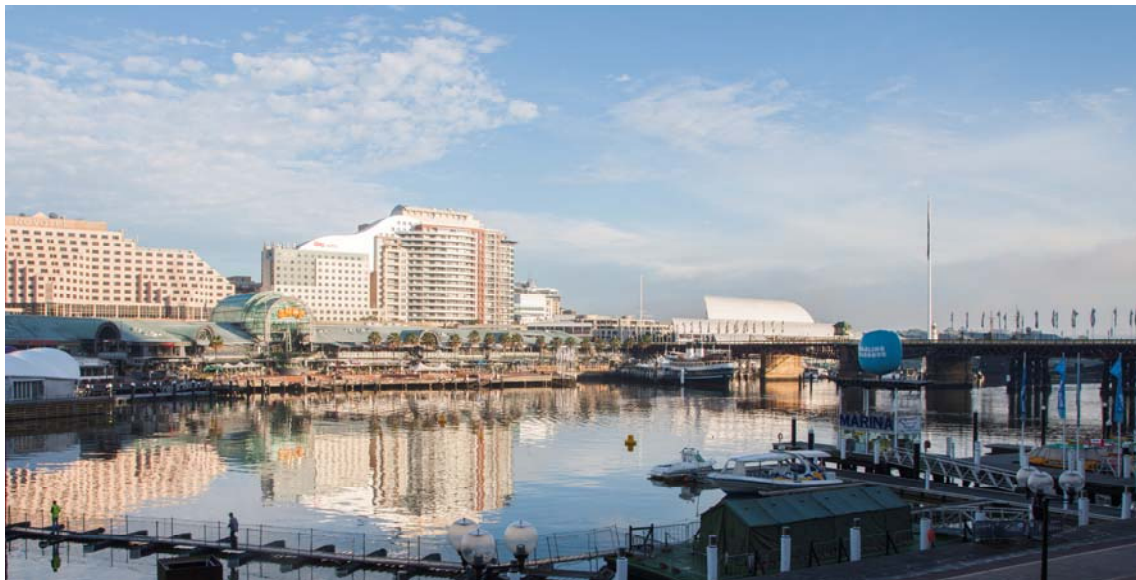
Figure 36: Before Renewal: Photo View East (Note structures in lower left corner are temporary event structures)
