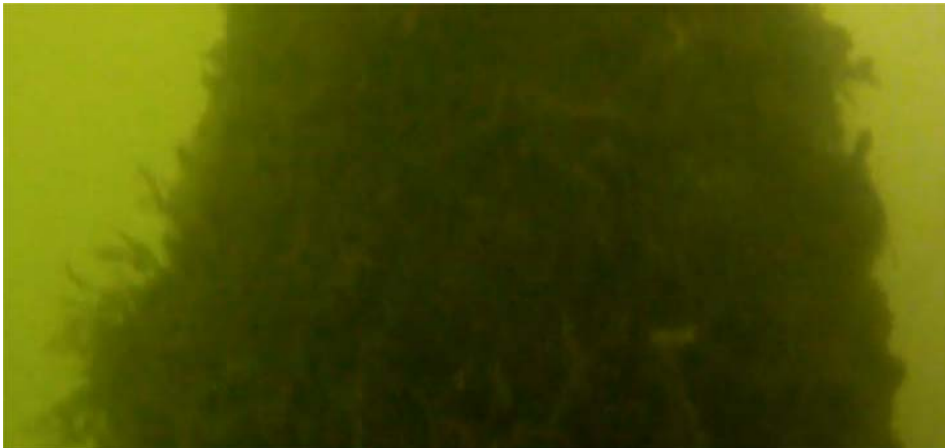
Figure 44: Dive Survey Footage of Aquatic Vegetation on Piles within the Project Area (Source: Cosmos Archaeology Pty Ltd, 2015)
