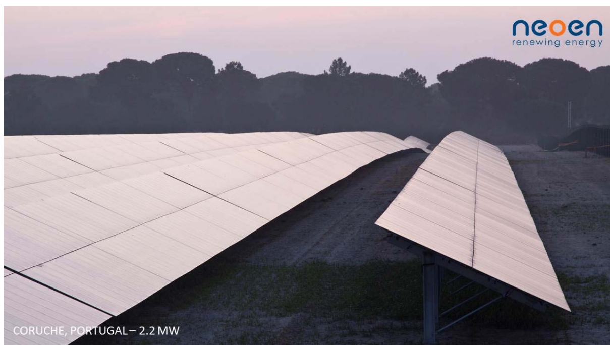
Figure 2-4 Example of south-facing fixed-tilt mounting system with thin-film technology in Europe (installation in Australia would face the north)
