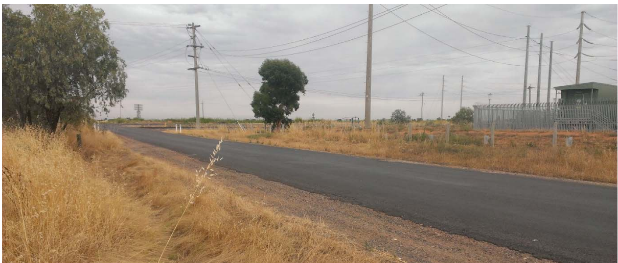
Figure 3-4 View of Hamilton Road and Transgrid substation
