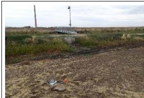
Plate 5. View east to IF1, note proximity of channel and water metre.
