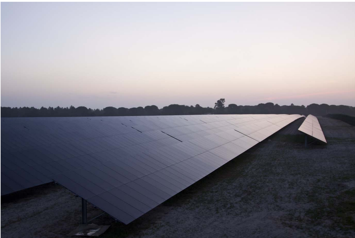
Figure 1-5 2.2MWp solar project constructed in Coruche, Portugal (Source Neoen Australia, 2014)
