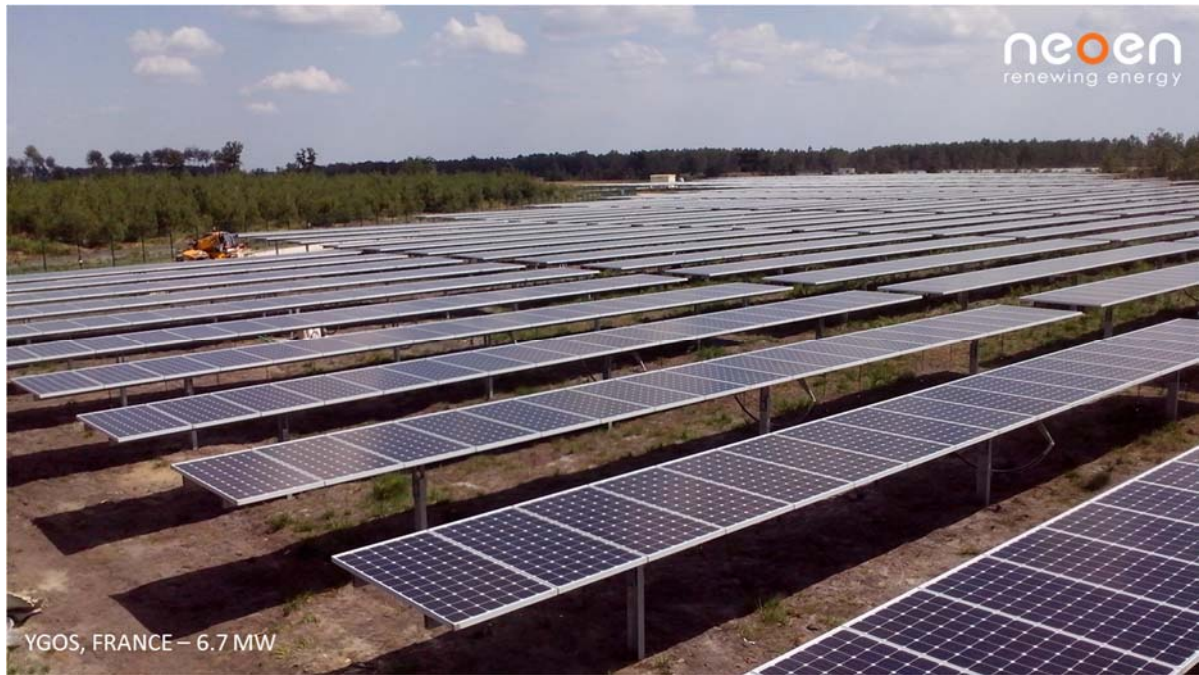
b) Operational array - Example of single-axis tracking systems with multicrystalline modules.
