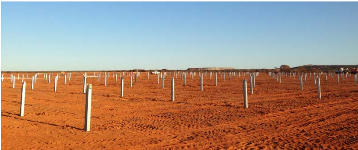
a) Driven piles, during construction.
