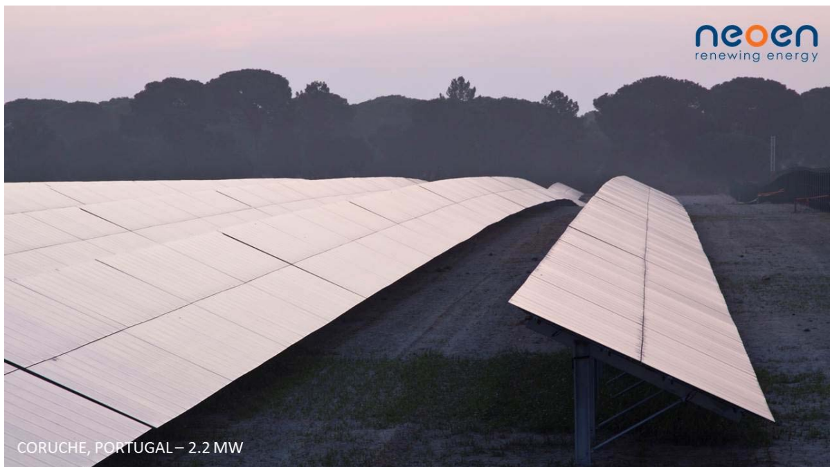
c) Example of north-facing fixed-tilt mounting system with thin-film technology.
