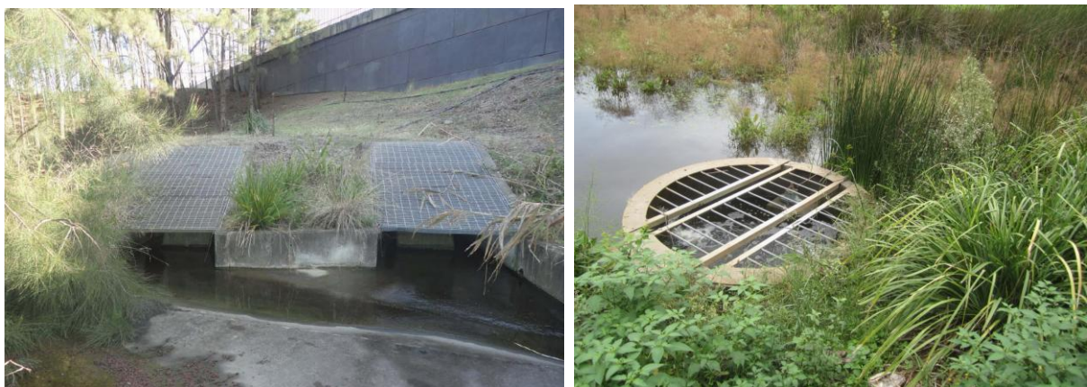
Figure 5: SWQCP inlet (L) and outlet (R) (Cardno 2012)
