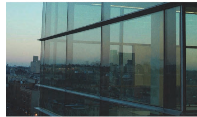
2. Double-glazed curtain wall facade system
