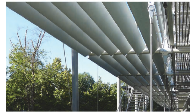
6. Anodized aluminium horizontal sun shades
