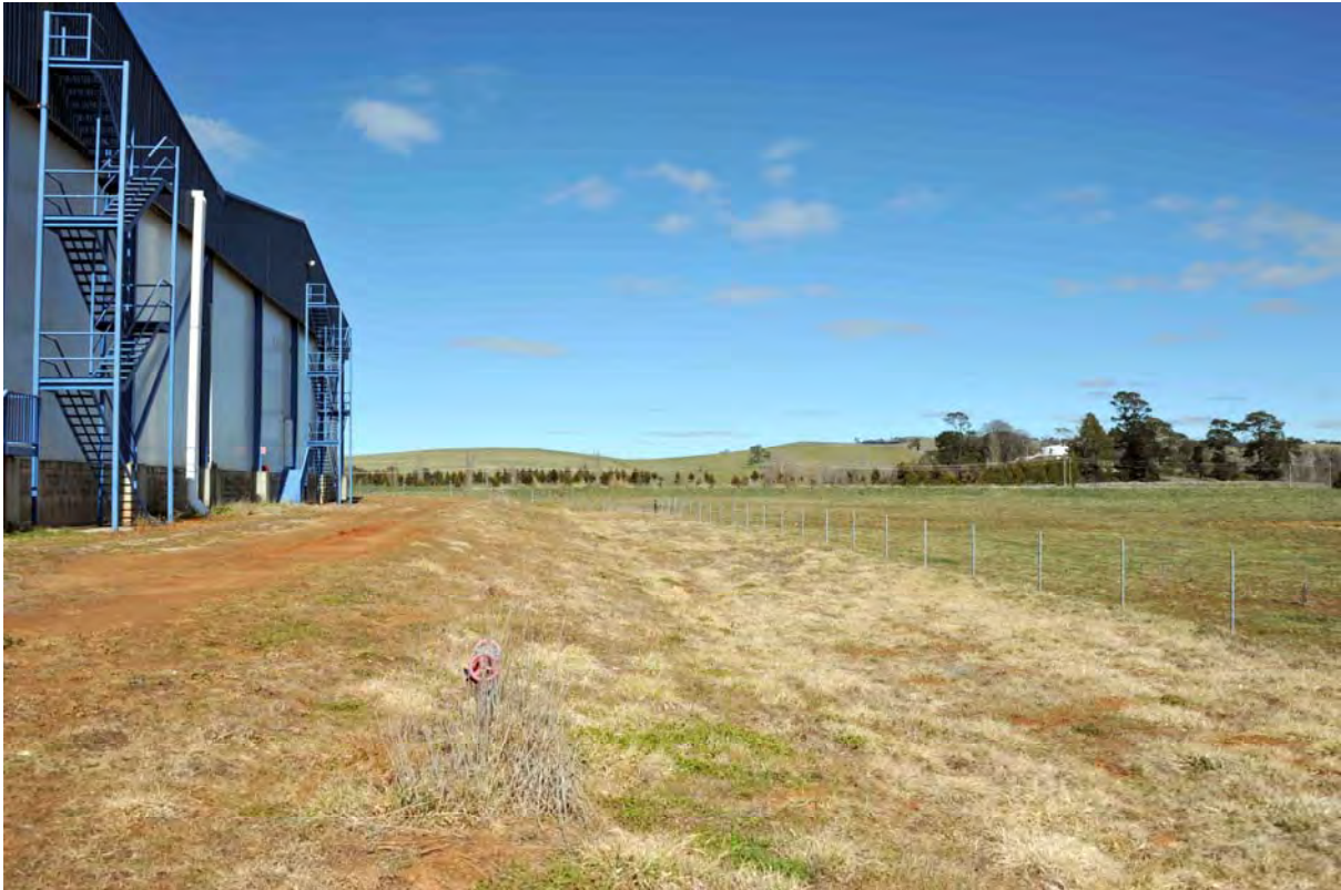
Plate 2 – View south across proposed abattoir site toward Newbridge Road and ‘Athol’ Homestead
