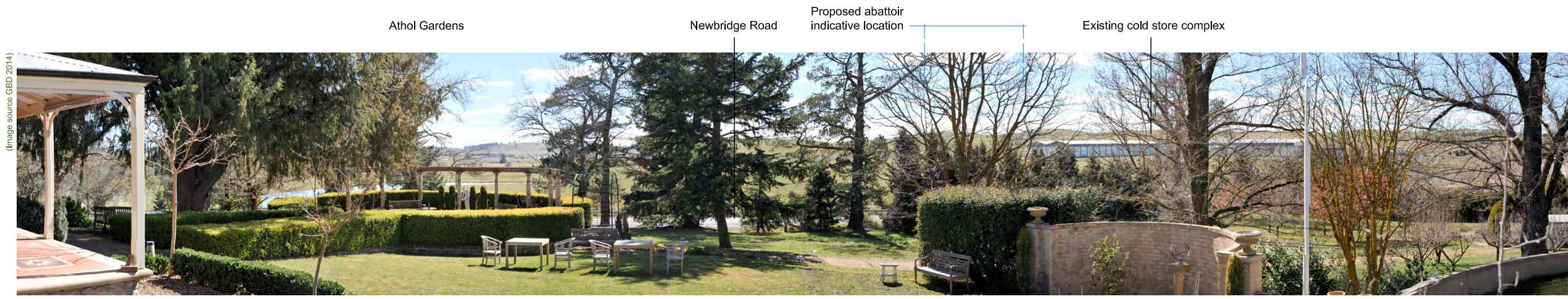
Photo Location A7 - View north to north west from Athol Gardens toward the existing cold store complex
