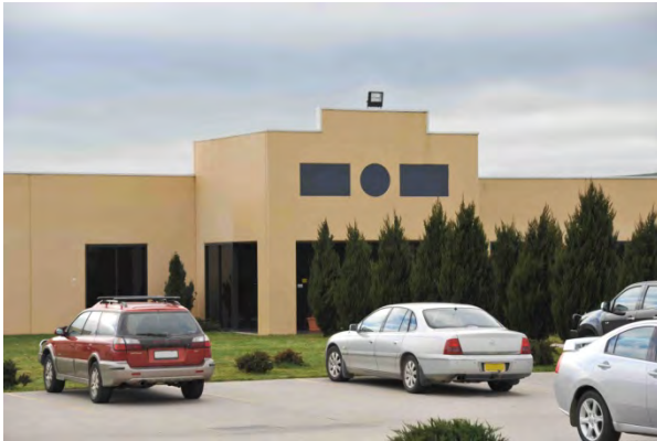
Plate 6 – Existing flood light on admin building
