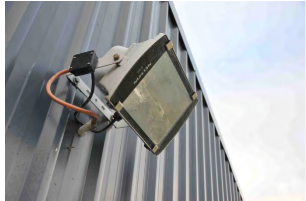
Plate 7 – Existing cold store external security lighting
