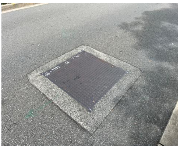
Figure 123 – Service pit in road pavement.
