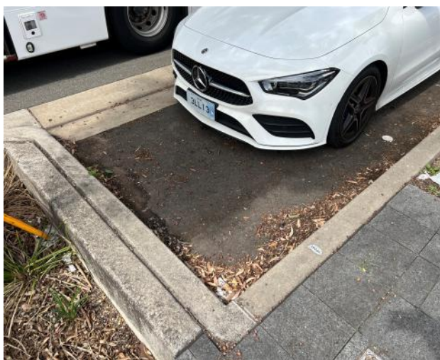
Figure 95 – Kerb and road pavement at parking bay.
