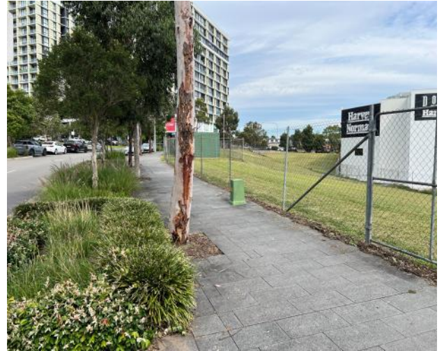
Figure 152 – General view of road pavement.
