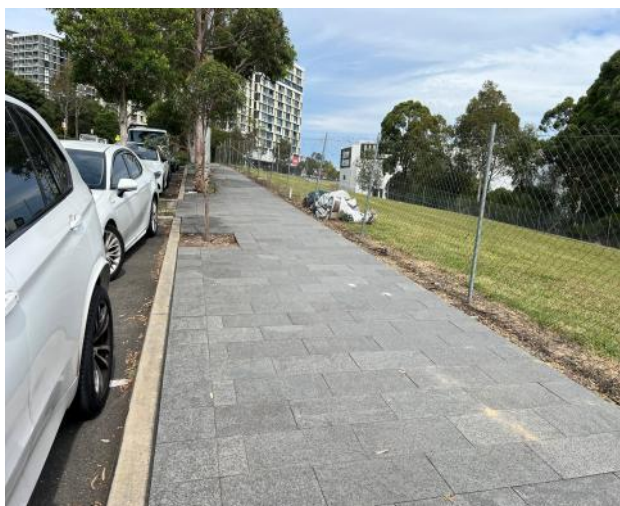
Figure 91 – General view of council footpath.
