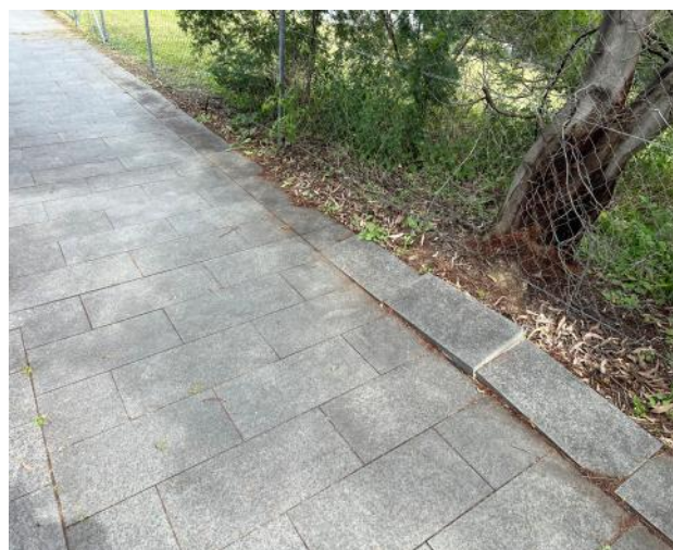
Figure 138 – General view of council footpath.
