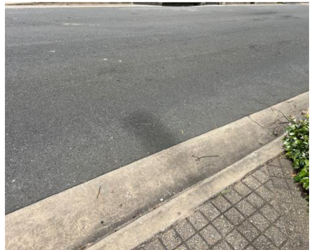
Figure 50 – General view of road pavement.
