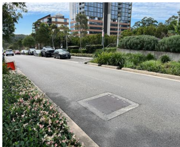
Figure 128 – General view of road pavement and service pit.
