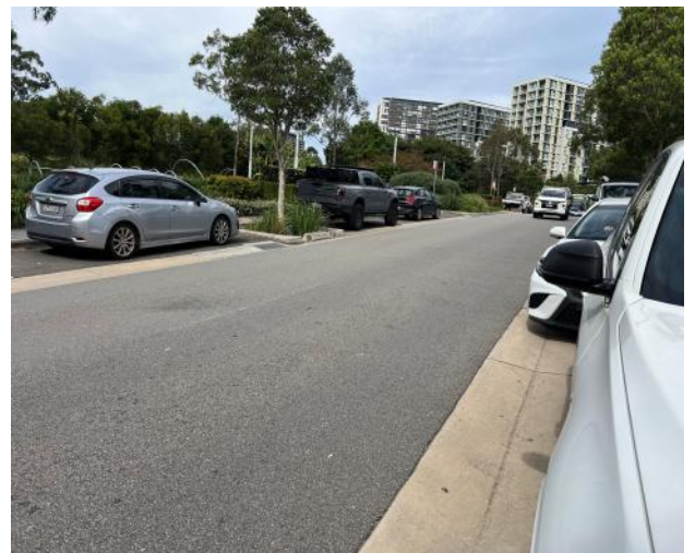
Figure 88 – General view of road pavement.
