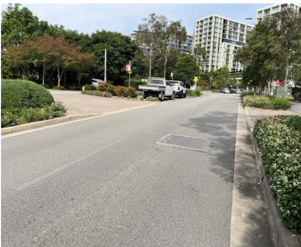
Figure 119 – General view of road pavement.
