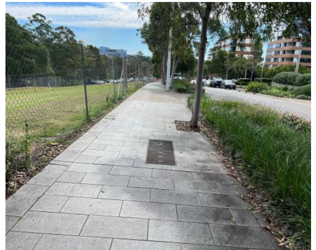
Figure 140 – General view of council footpath.
