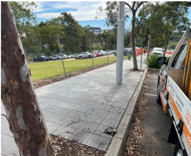
Figure 25 – General view of footpath and power pole.
