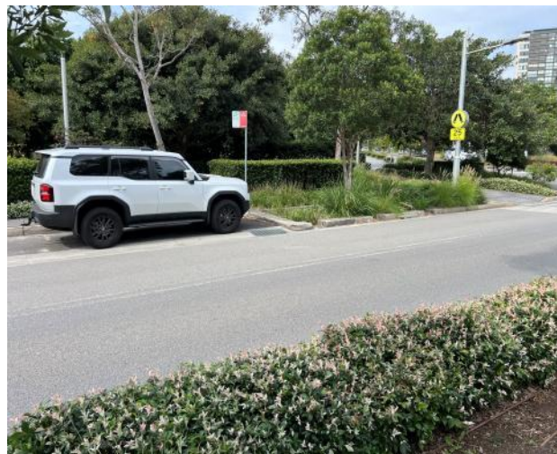
Figure 134 – General view of road pavement.
