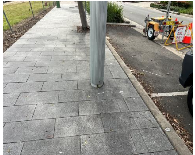
Figure 26 – General view of base of power pole.
