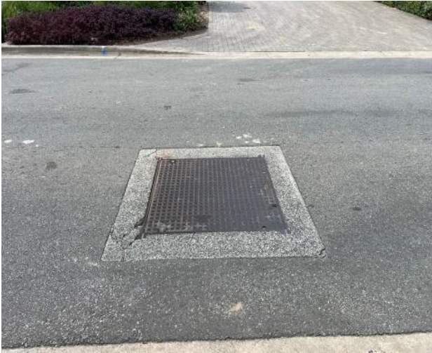
Figure 61 – General view of service pit.
