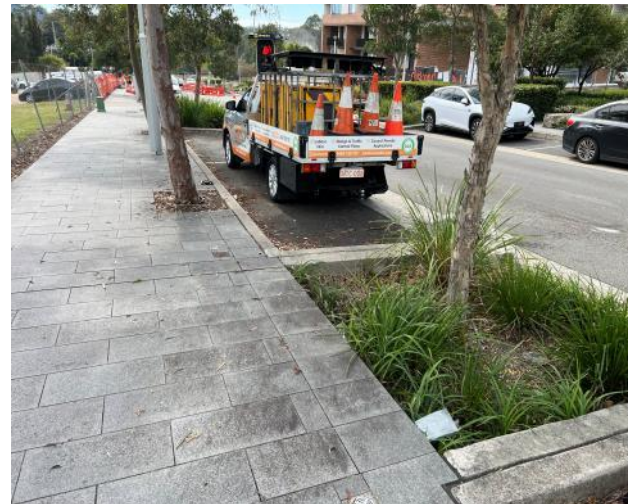
Figure 2 – General view of council footpath.
