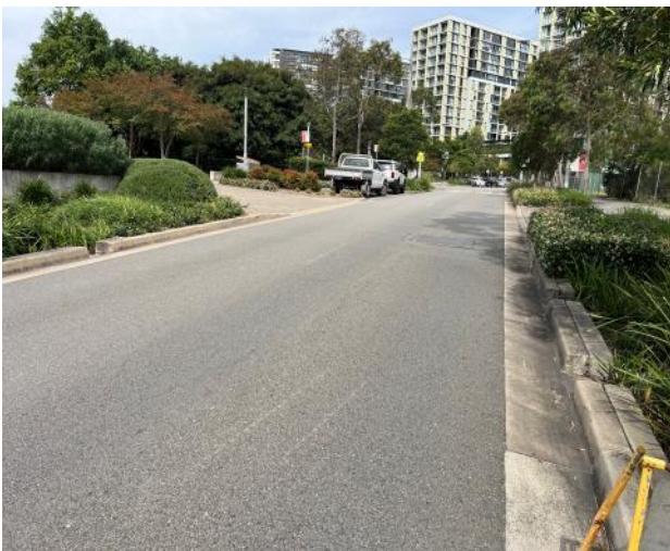
Figure 117 – General view of road pavement.
