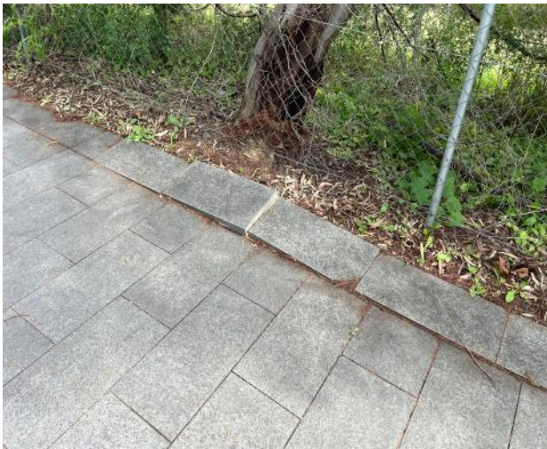
Figure 139 – General view of council footpath.
