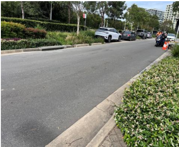
Figure 49 – General view of road pavement.
