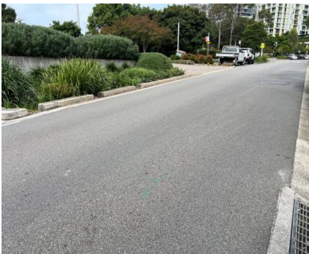
Figure 113 – General view of road pavement.
