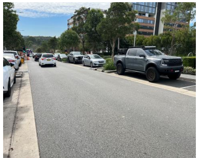
Figure 108 – General view of road pavement.
