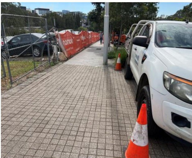
Figure 47 – General view of council footpath.
