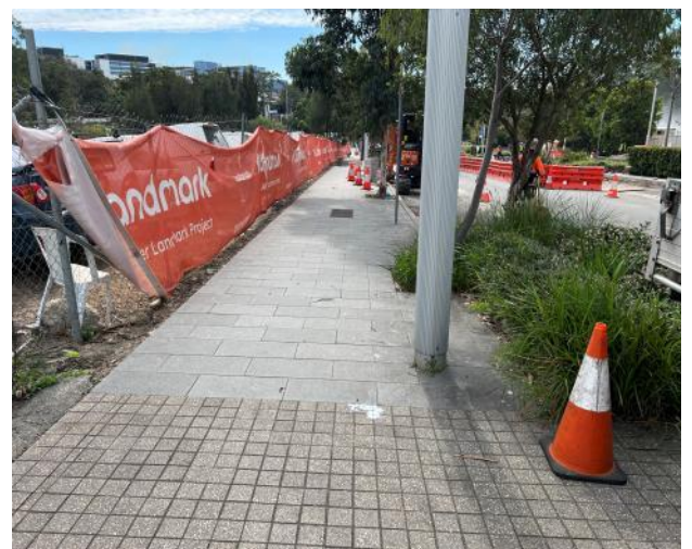
Figure 60 – General view of council footpath.
