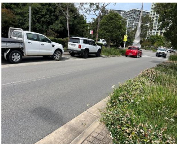
Figure 131 – General view of road pavement.
