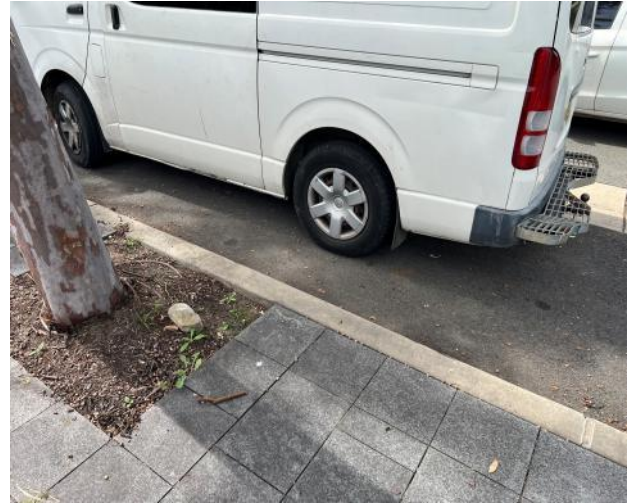
Figure 104 – kerb and road pavement.
