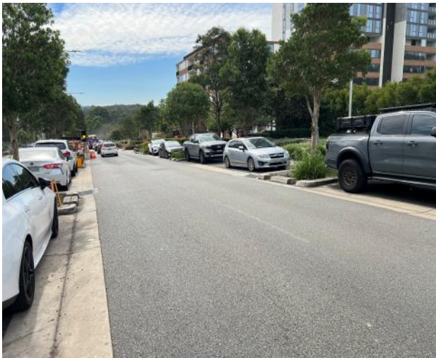
Figure 109 – General view of road pavement.
