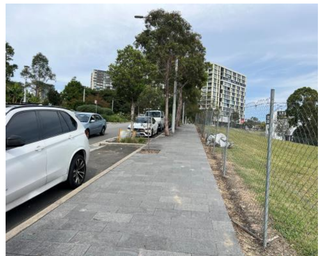
Figure 84 – General view of council footpath.
