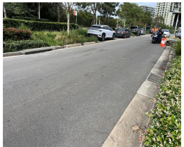
Figure 52 – General view of road pavement.
