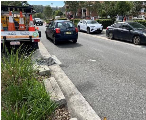
Figure 19 – General view of road pavement.
