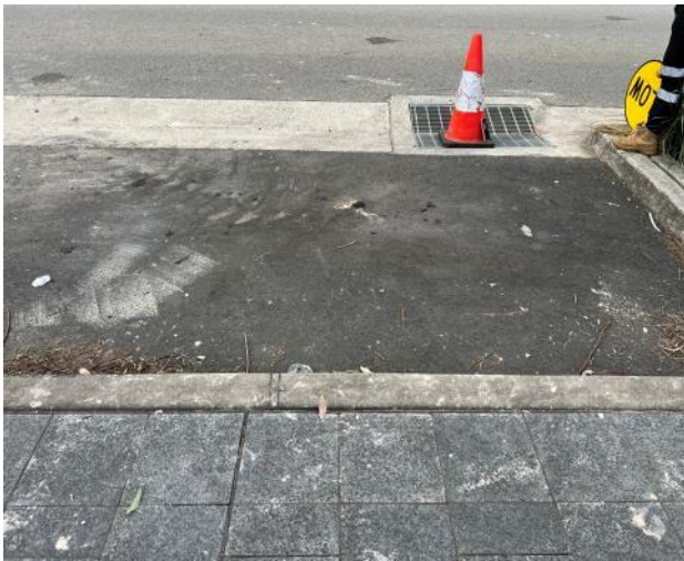
Figure 73 – General view of parking bay.
