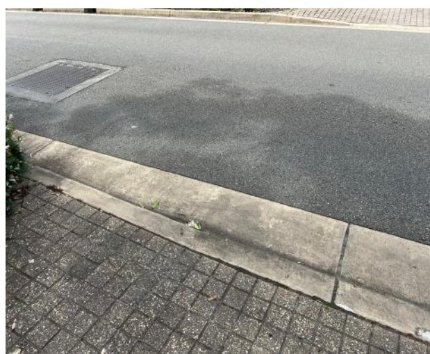
Figure 130 – General view of road pavement, kerb and gutter.
