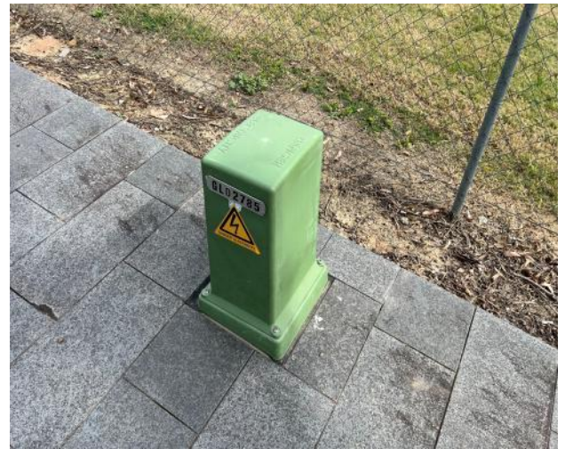
Figure 44 – Current condition of electrical pit/box.
