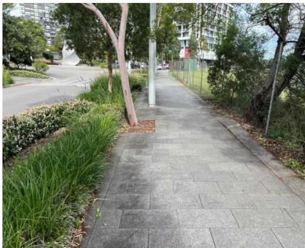
Figure 133 – General view of council footpath.
