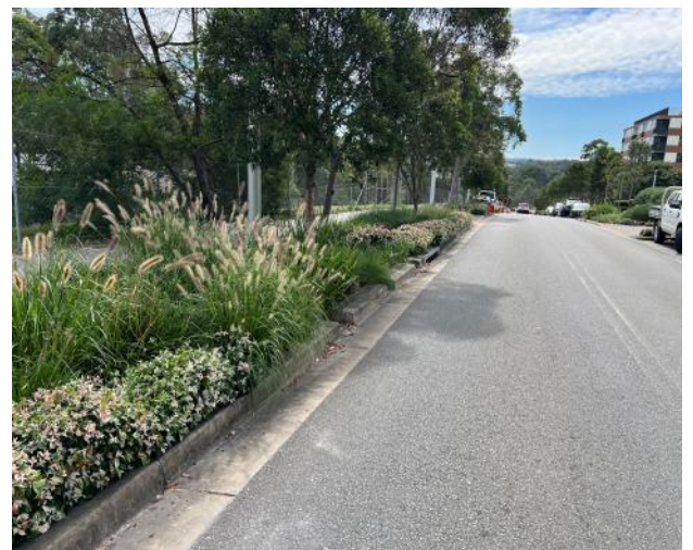
Figure 150 – General view of road pavement, kerb and gutter.
