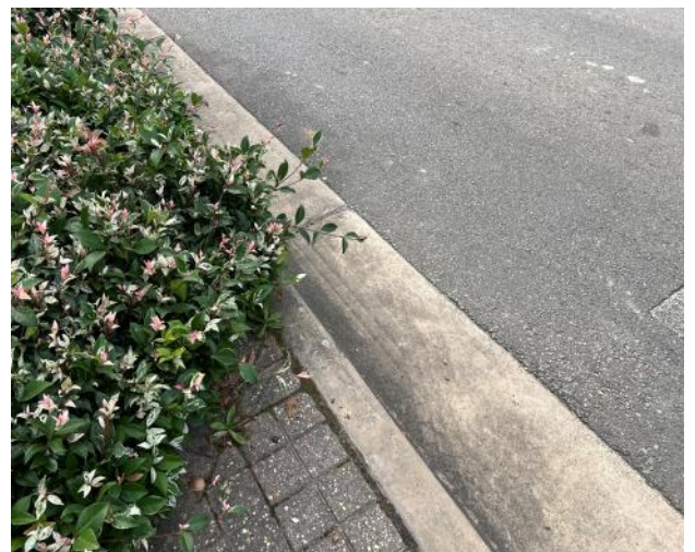
Figure 66 – Kerb and gutter.
