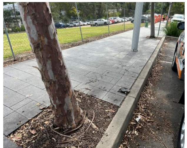
Figure 24 – General view of tree and kerb on council land.
