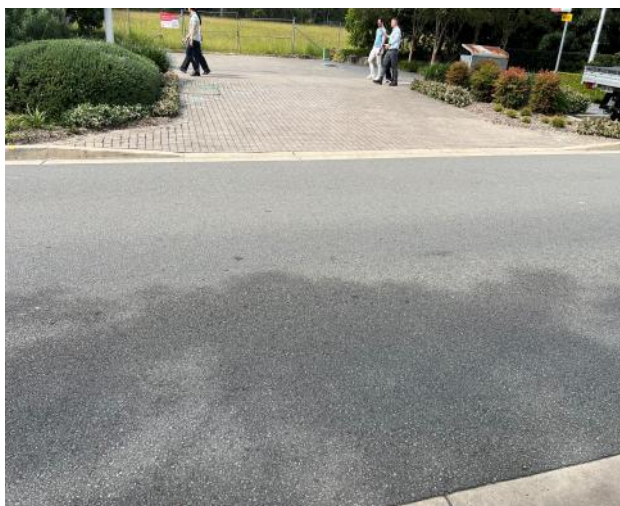
Figure 127 – General view of road pavement.
