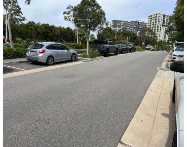
Figure 14 – General view of road pavement.
