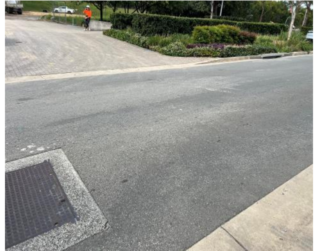
Figure 62 – General view of road pavement.
