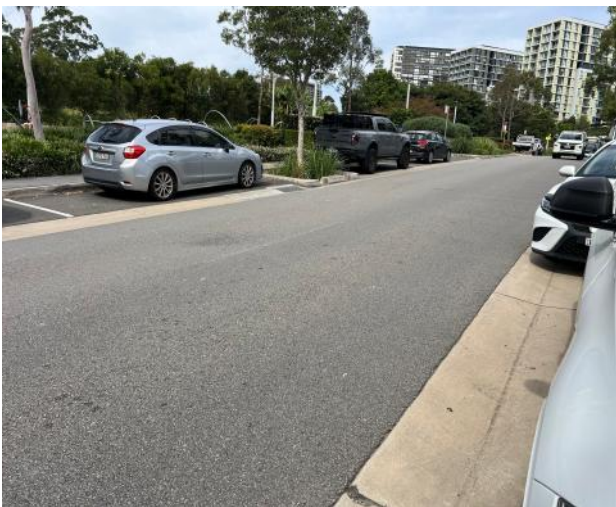
Figure 87 – General view of road pavement.
