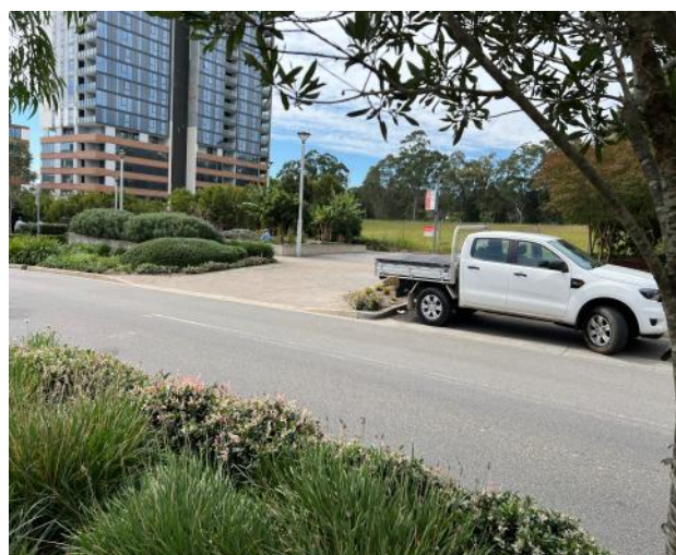
Figure 136 – General view of road pavement.
