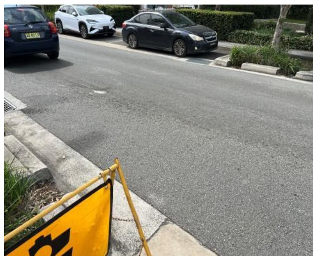
Figure 12 – General view of road pavement.
