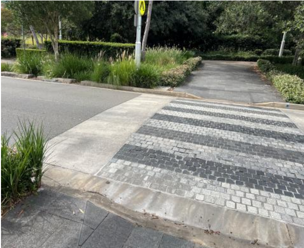
Figure 145 – General view of road crossing.
