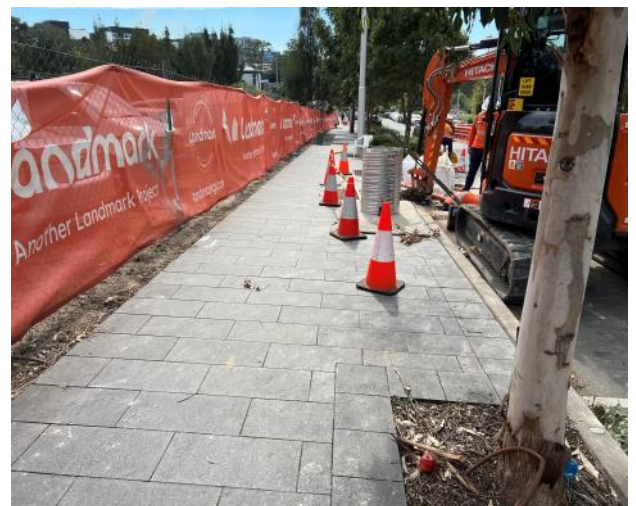
Figure 78 – General view of council footpath.
