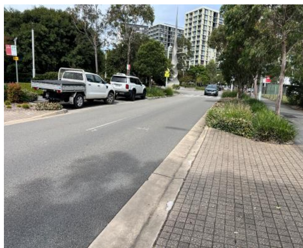
Figure 126 – General view of road pavement.
