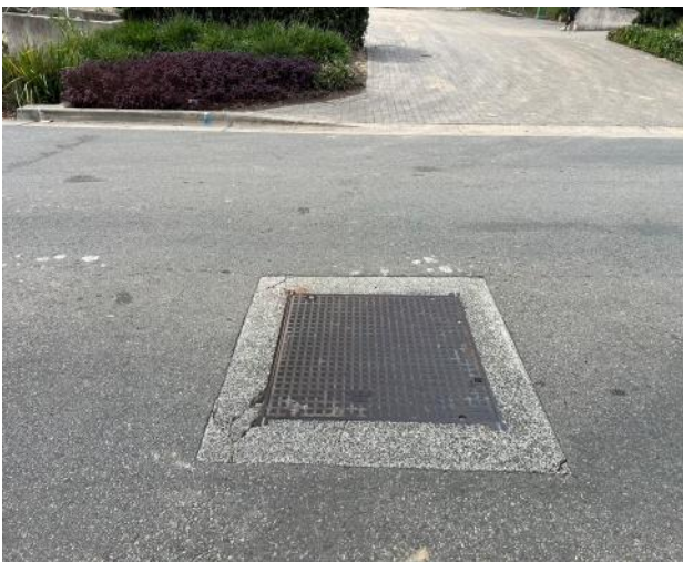
Figure 63 – General view of service pit.
