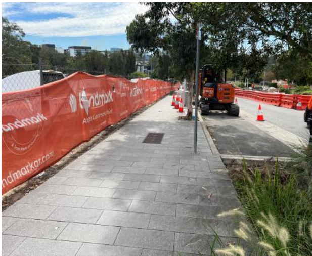
Figure 67 – General view of council footpath.
