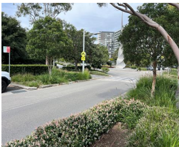
Figure 135 – General view of road pavement.
