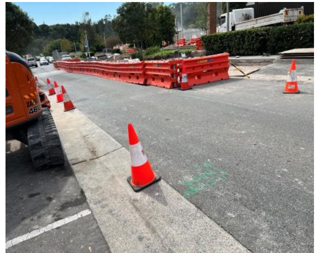
Figure 74 – General view of road pavement.
