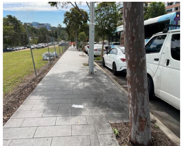
Figure 106 – General view of council footpath.
