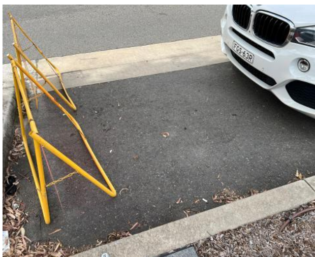
Figure 11 – General view of road pavement at parking bay.
