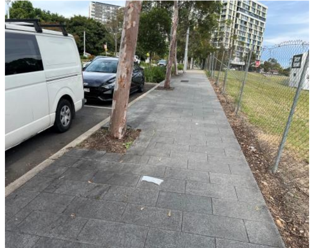
Figure 98 – General view of council footpath.
