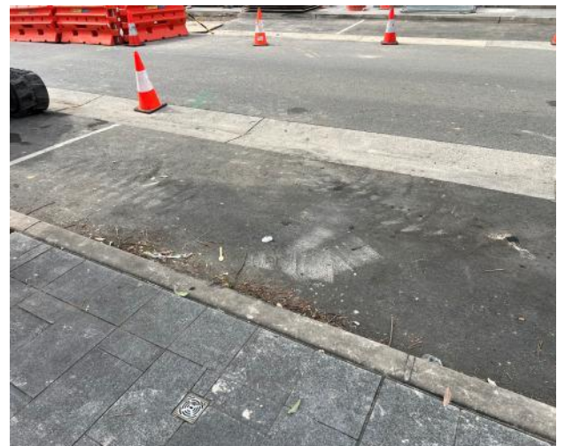
Figure 72 – General view of road pavement.
