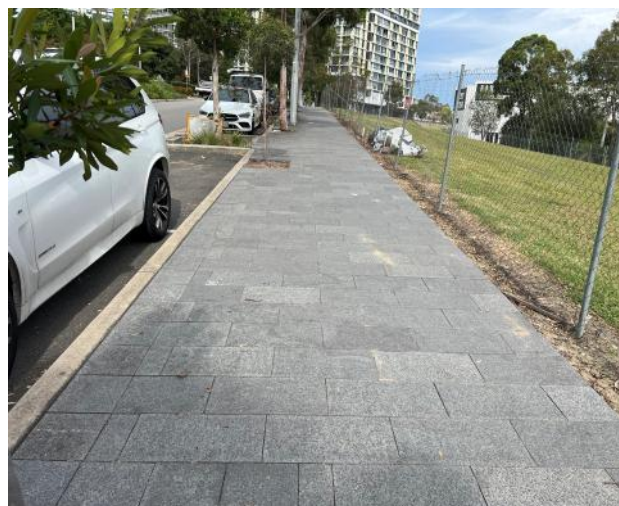
Figure 8 – General view of council footpath.
