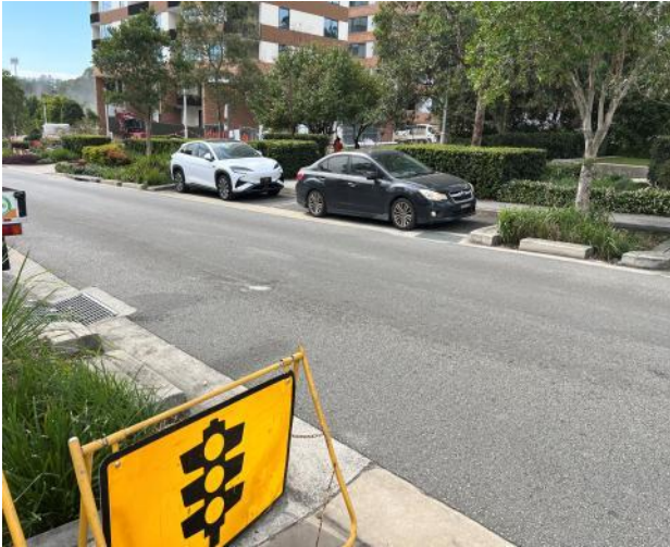
Figure 85 – General view of road pavement.
