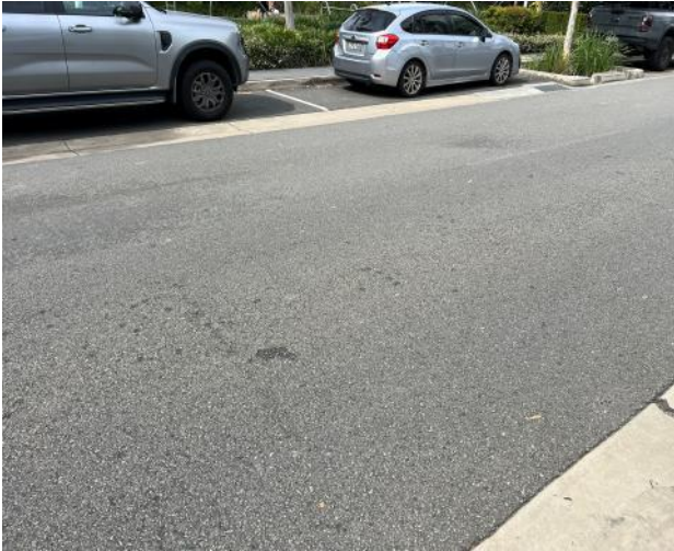
Figure 13 – General view of road pavement.
