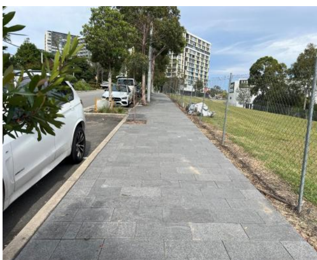
Figure 9 – General view of council footpath, kerb and gutter.
