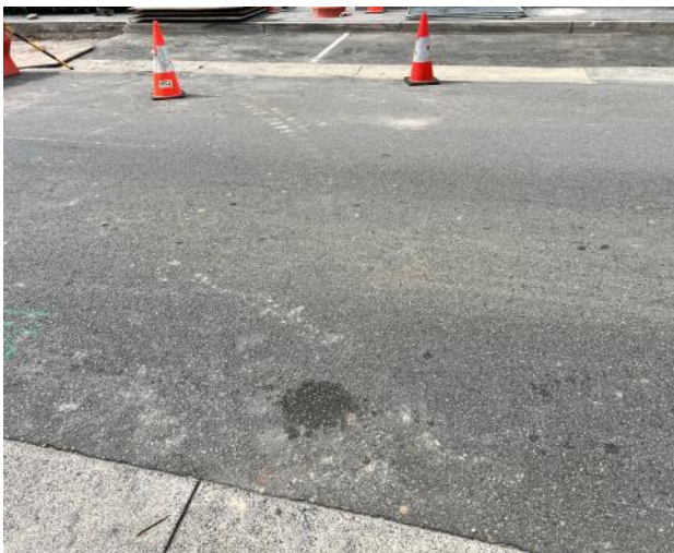
Figure 75 – General view of road pavement.
