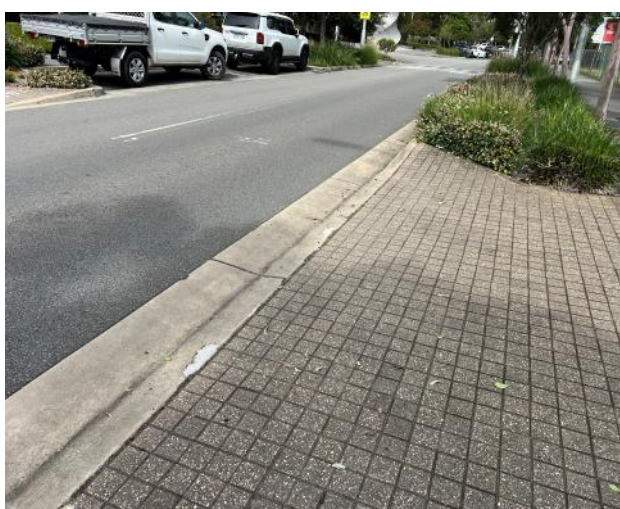
Figure 129 – General view of road pavement, kerb and gutter.
