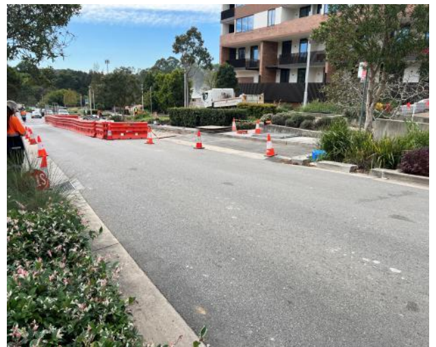
Figure 64 – General view of road pavement.
