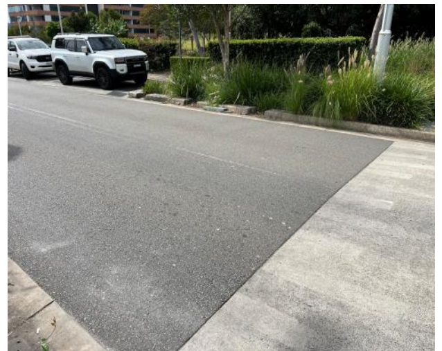
Figure 148 – General view of road pavement.
