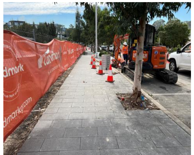
Figure 70 – General view of council footpath.
