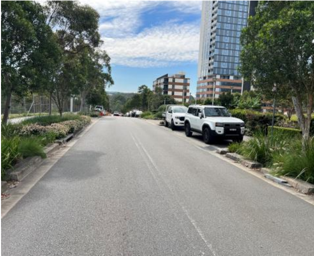
Figure 151 – General view of road pavement.
