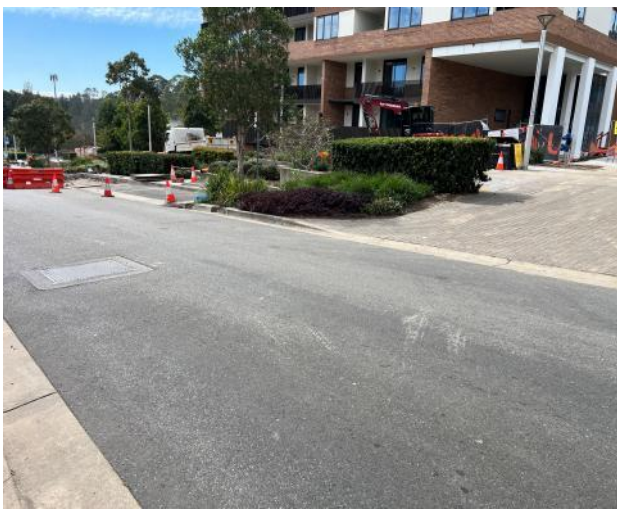
Figure 57 – General view of road pavement.
