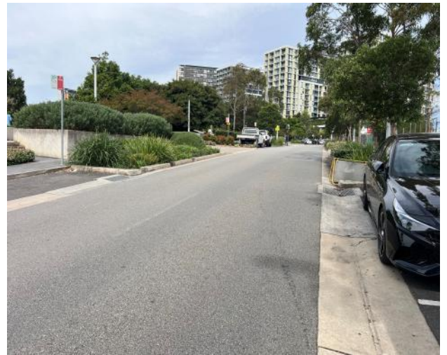
Figure 110 – General view of road pavement.
