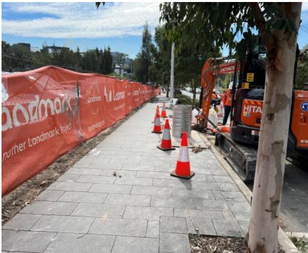
Figure 79 – General view of council footpath.
