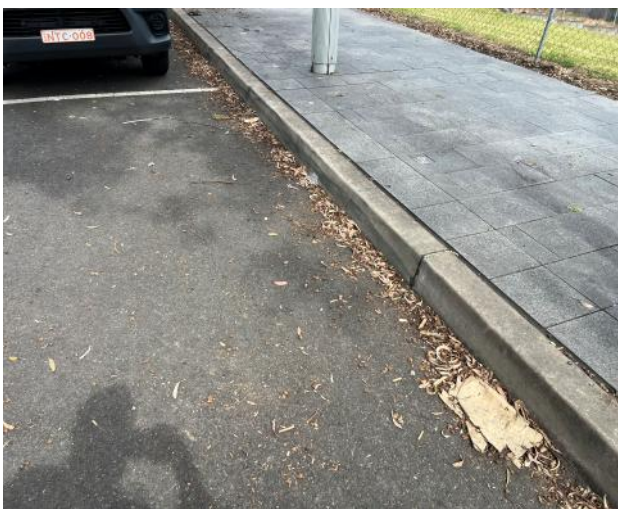
Figure 33 – General view of kerb.
