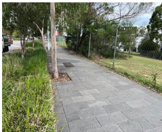
Figure 132 – General view of council footpath.
