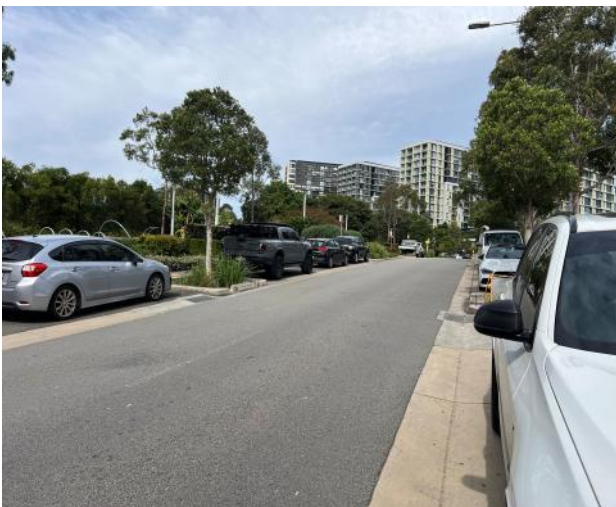
Figure 15 – General view of road pavement.
