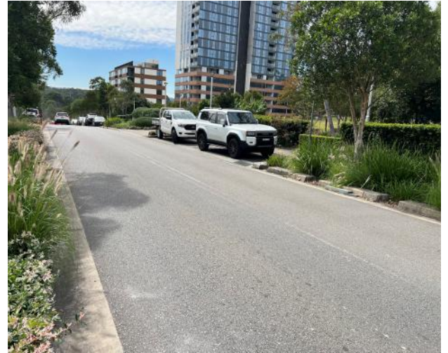
Figure 146 – General view of road pavement.
