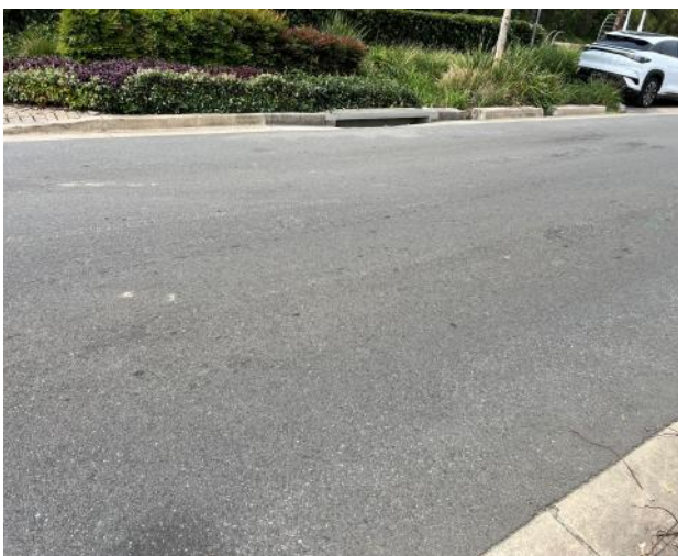
Figure 53 – General view of road pavement.
