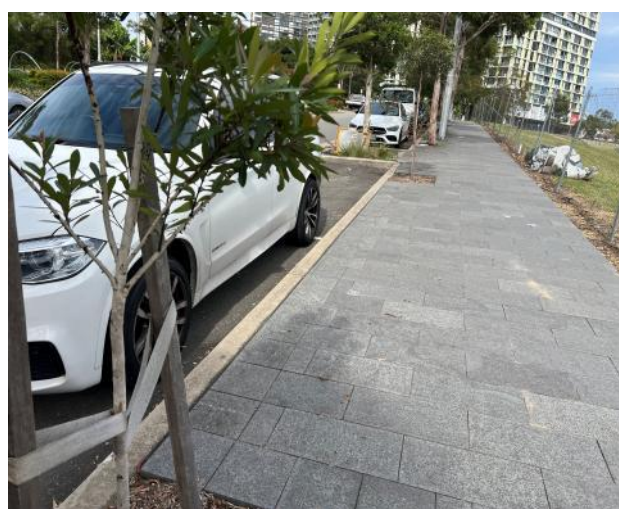
Figure 10 – General view of footpath and kerb.
