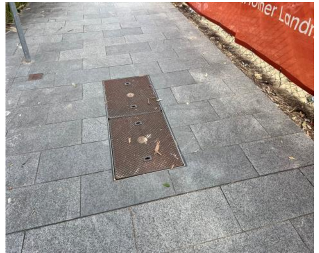
Figure 80 – General view of service pit.
