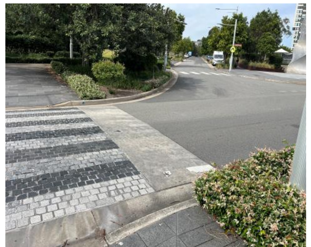
Figure 144 – General view of road crossing.
