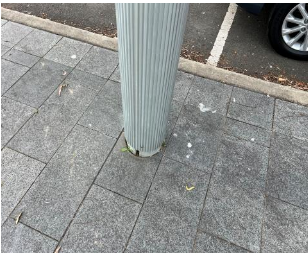
Figure 27 – General view of base of power pole.
