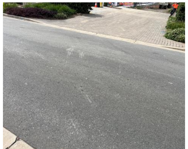
Figure 54 – General view of road pavement.
