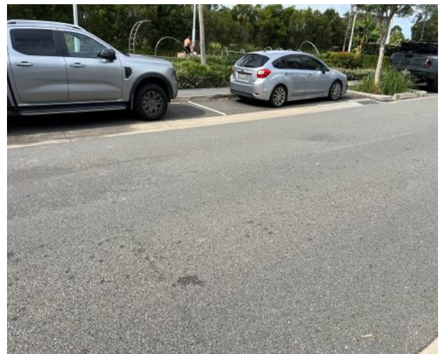
Figure 16 – General view of road pavement.
