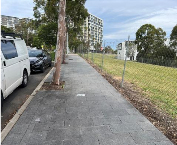
Figure 97 – General view of council footpath.
