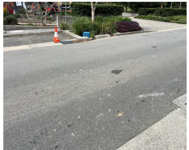
Figure 76 – General view of road pavement.
