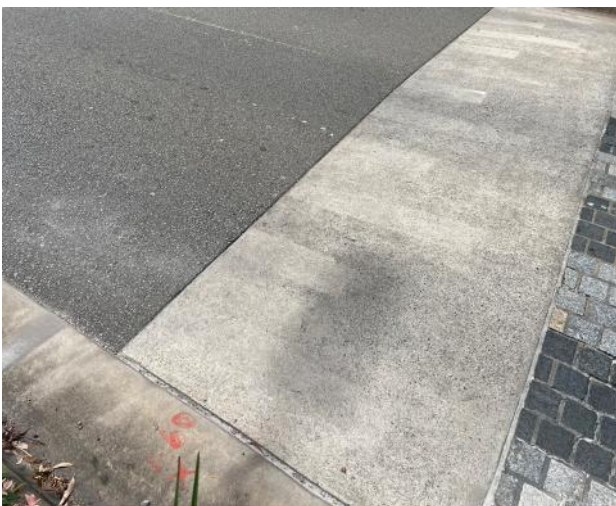
Figure 149 – General view of road pavement.
