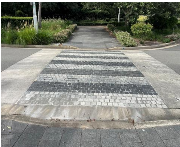
Figure 143 – General view of road crossing.
