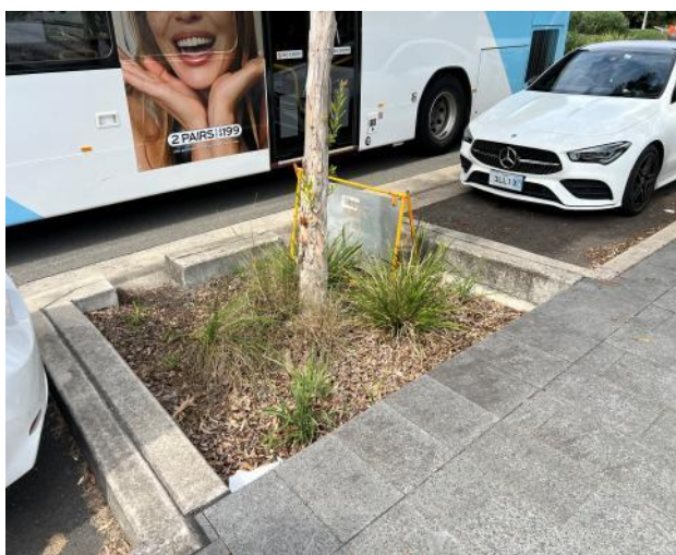
Figure 93 – General view of council tree pit.
