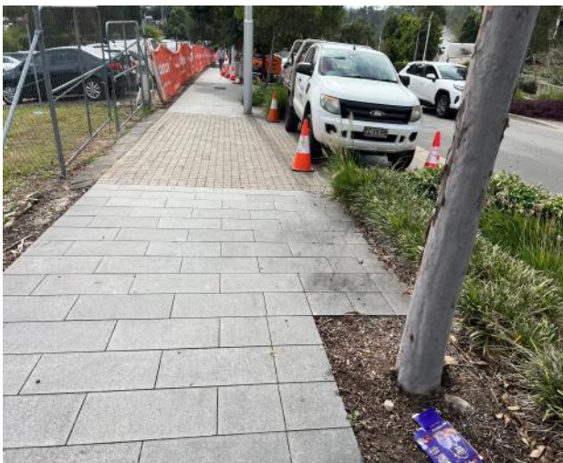
Figure 45 – General view of council footpath.
