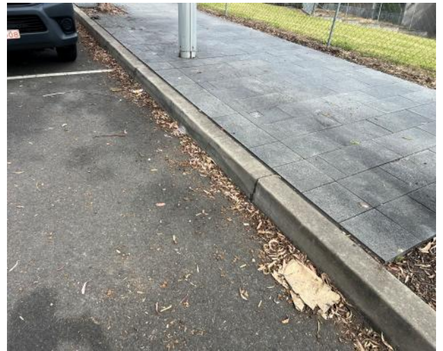
Figure 32 – kerb and council road pavement.
