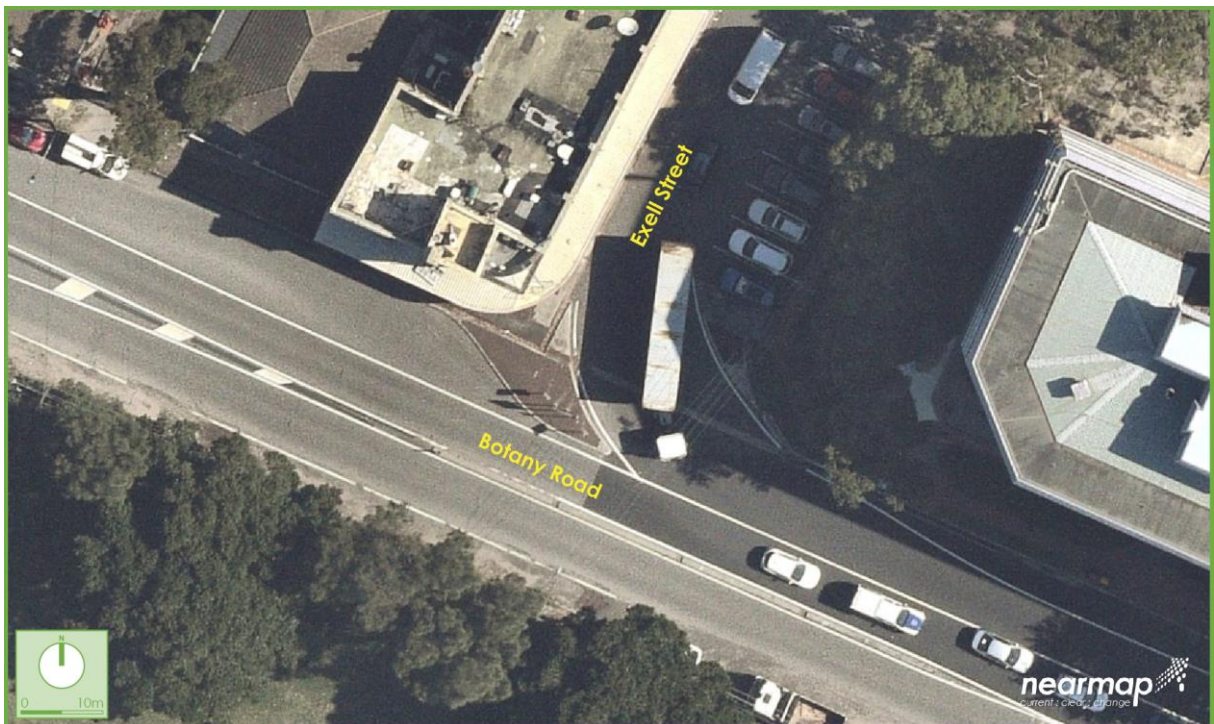
Figure 5: Intersection of Botany Road and Exell Street
