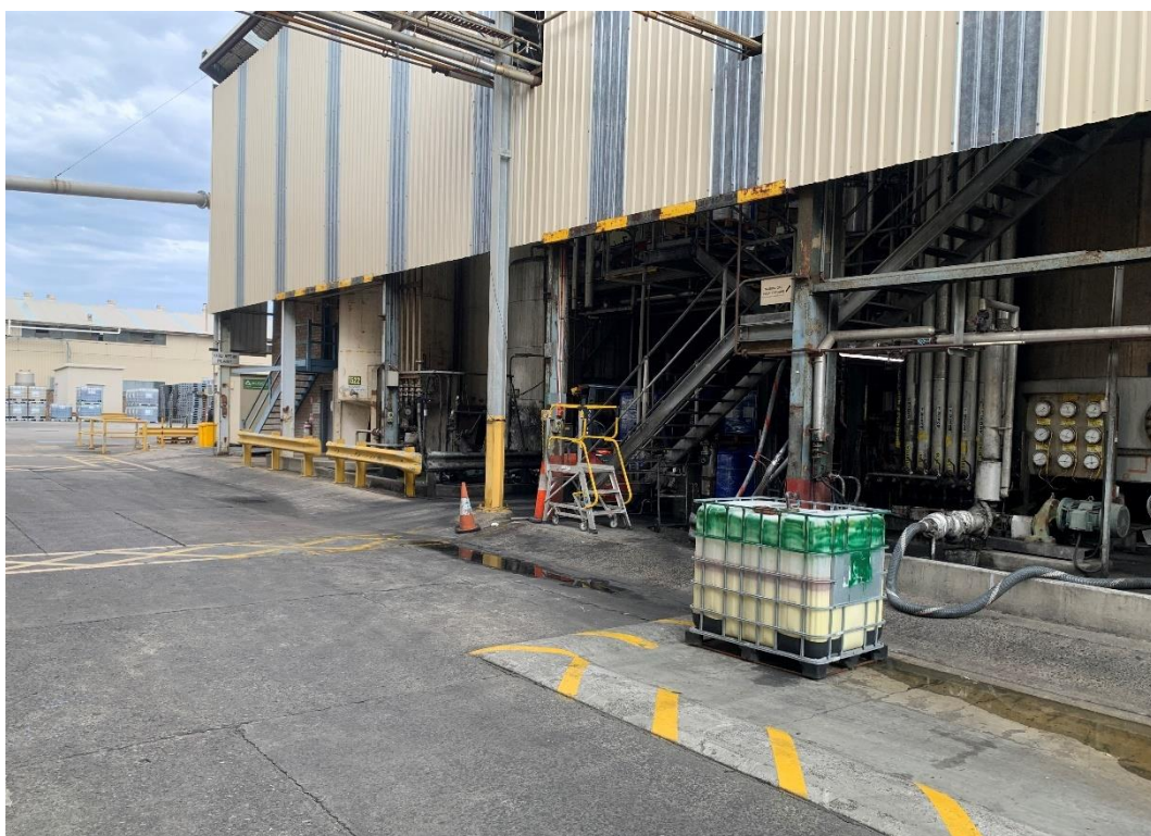
Photo 76: Hard Resin Plant Building - Blending Plant (Looking South-East)
