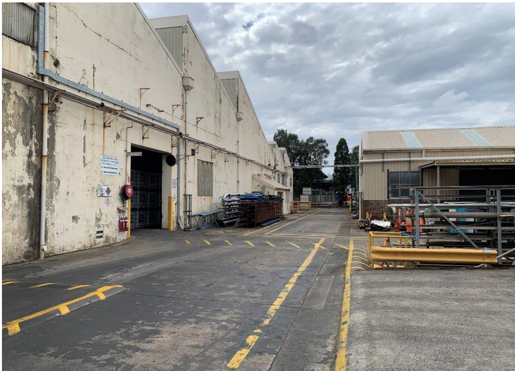
Photo 92: Looking North Between the Emulsions Plant Storage Building and Engineering Workshop
