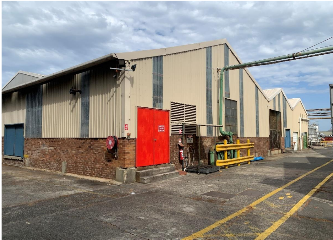
Photo 93: Fire Sprinkler and Hydrant Pump Room
