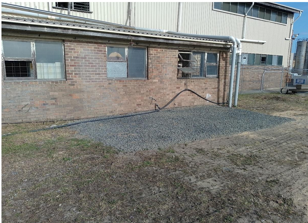
Photo 117: Nuodex Plant Spill Area Backfilled and Covered with Plastic and Gravel
