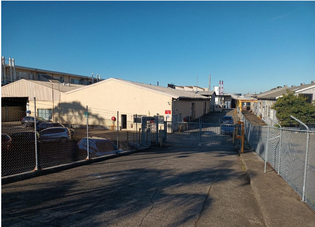
Photo 13: Access Ramp to Staff Car Park (Looking East Along Southern Boundary from Stephen Road)
