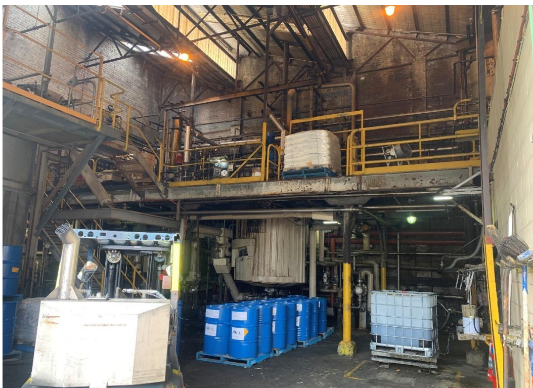
Photo 78: Hard Resin Plant Building
