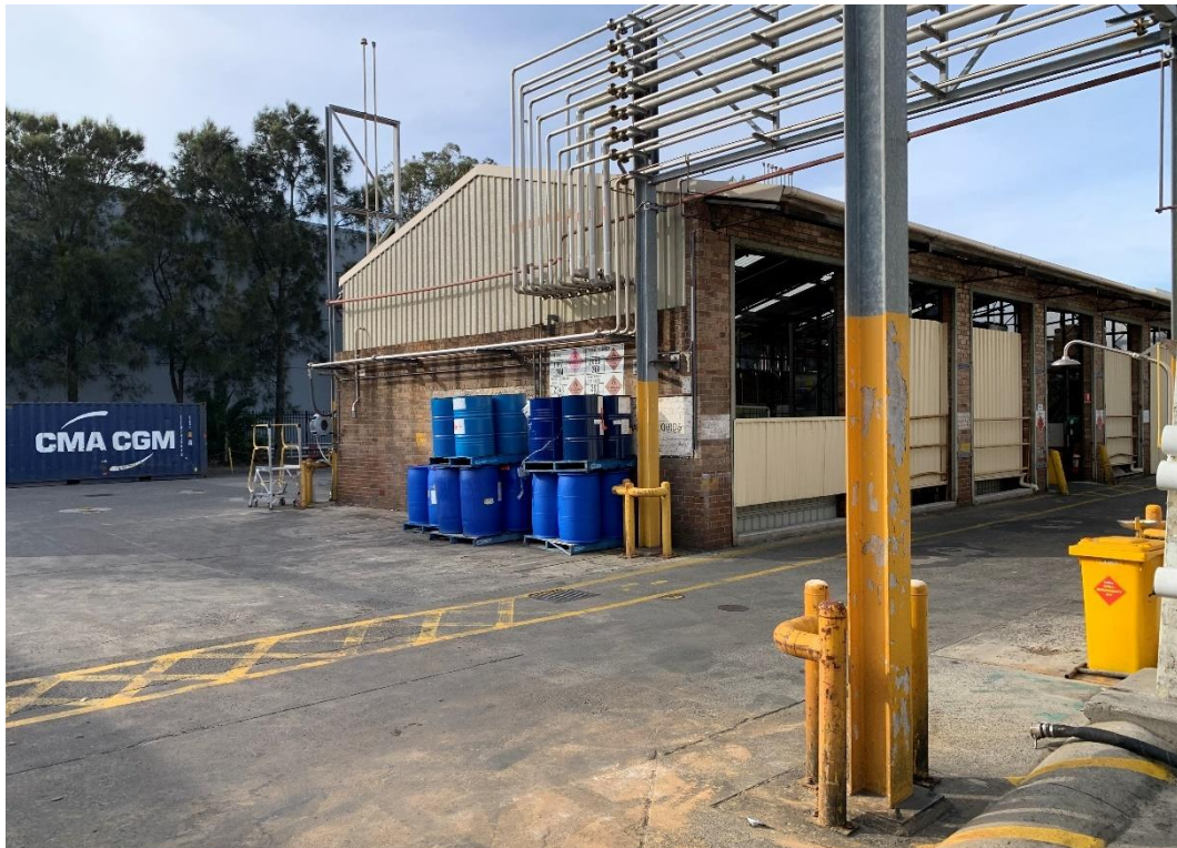
Photo 35: Area of Redundant UST Adjacent to the Northern UST Pump Room
