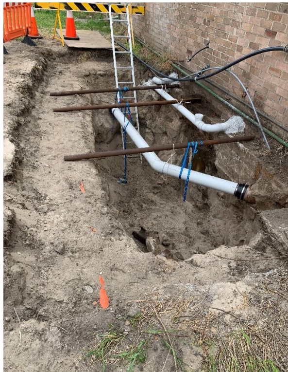
Photo 116: Nuodex Plant Spill Area Initial Excavation - Eastern Grass Area
