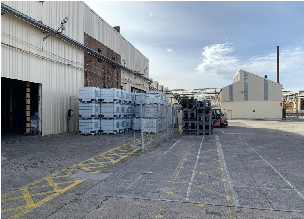
Photo 83: Storage and Truck Loading Area East of the Hard Resin Plant Building
