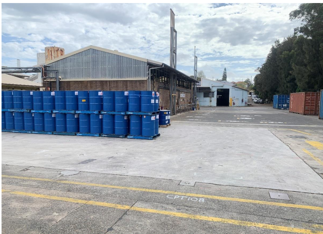
Photo 30: Northern UST Farm and Associated Pump Room and Loading Area (Looking West)
