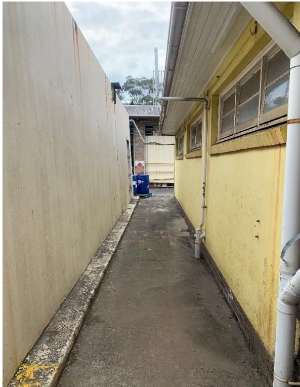
Photo 37: Eastern Side of the Central AST Farm (Looking North Towards BH336)
