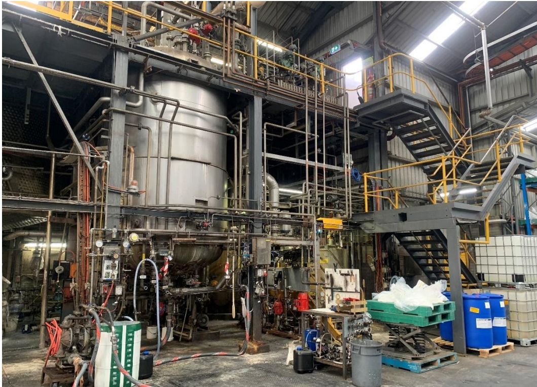
Photo 43: Emulsions Plant Building (East)
