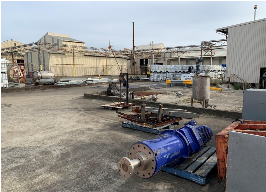
Photo 102: Storage Area and Eastern Car Park (Looking South-West)
