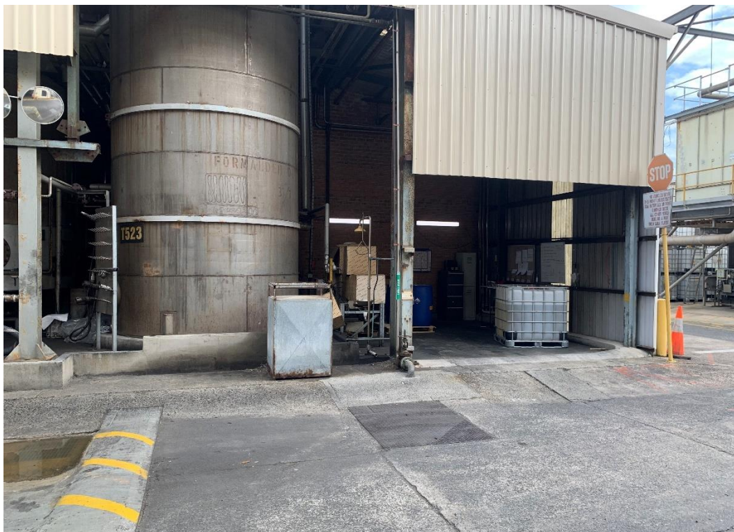
Photo 77: Hard Resin Plant Building - Blending Plant (West)
