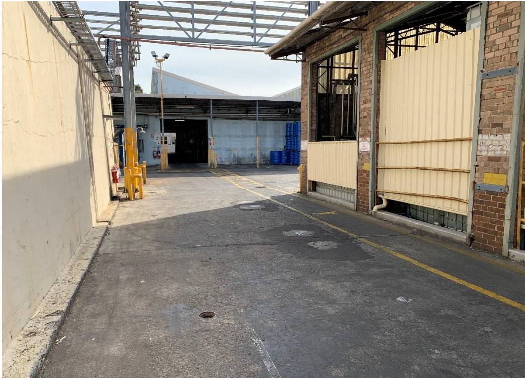
Photo 34: Area of Redundant UST Adjacent to the Northern UST Pump Room
