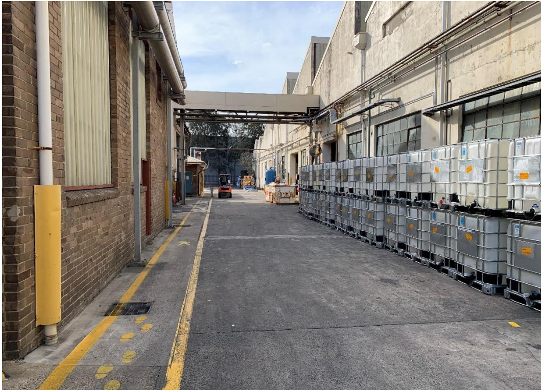
Photo 45: Between Emulsions Plant and Storage Buildings (Looking North)
