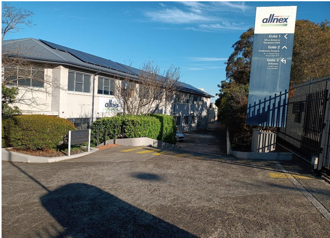
Photo 1: Administration Building and Ramp Down to Car Parking Area
