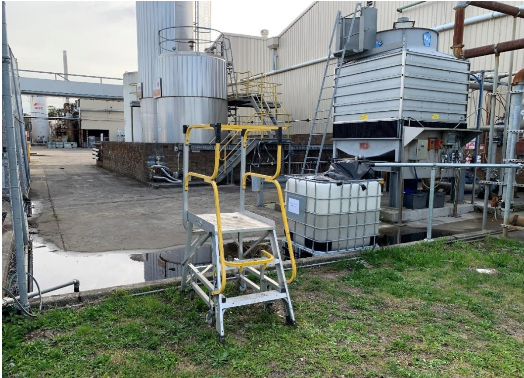
Photo 113: South-East (Nuodex Plant) AST Farm (Looking West)
