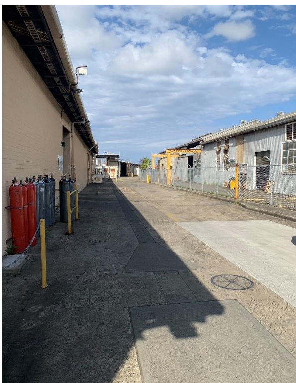
Photo 66: Boundary Remediation System and Southern Boundary (Looking East)
