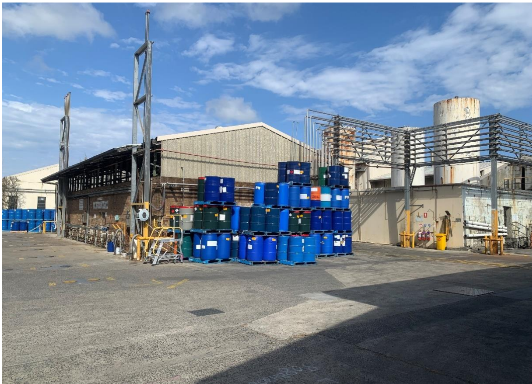
Photo 32: North UST Farm Pump Room Building, Loading Area and Area of Redundant USTs
