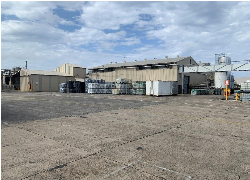
Photo 90: Truck Loading Area (Looking North-East Towards Nuodex Plant)
