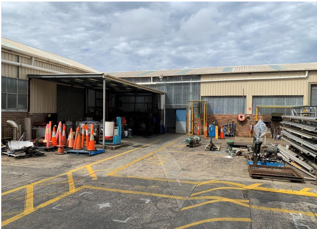
Photo 96: Engineering Workshop External Area (Looking East)
