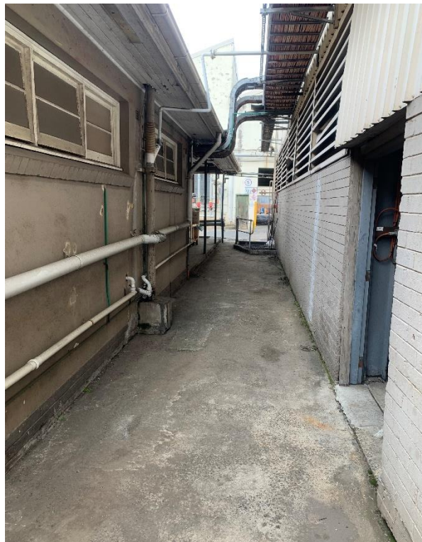
Photo 40: Corridor Between Emulsions Plant Control Room and Production Buildings
