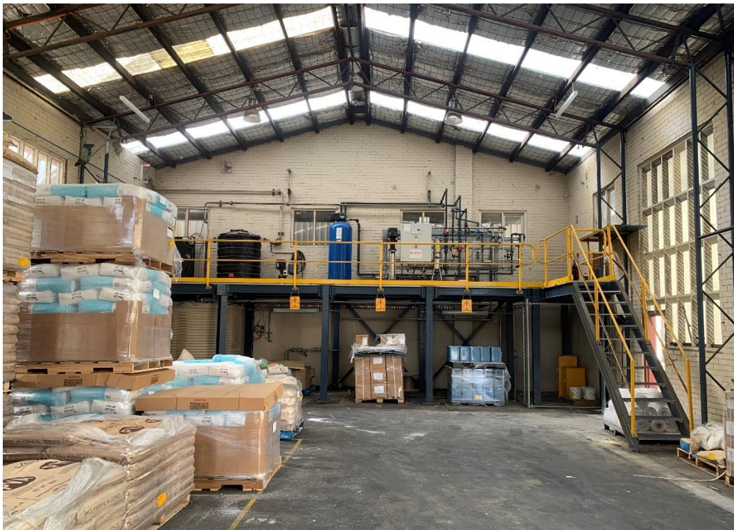
Photo 56: Brick Building - Storage and Water Plant Room
