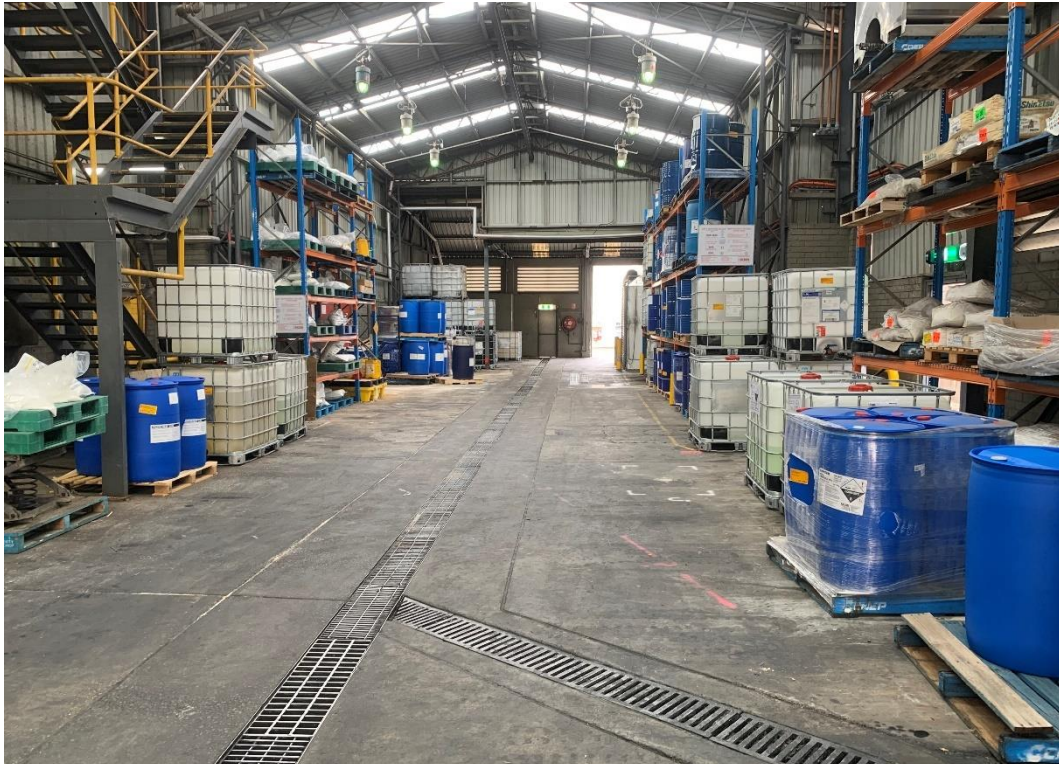
Photo 41: Emulsions Plant Building (Looking West)
