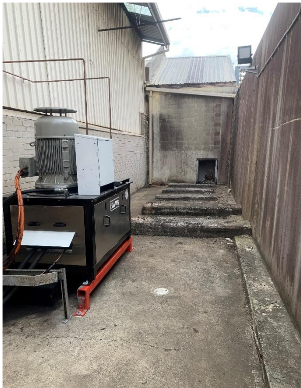
Photo 38: South Side of the Central AST Farm
