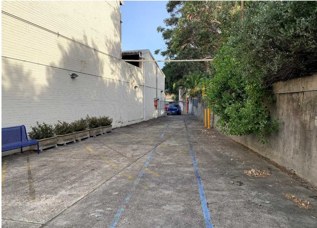
Photo 3: Car Parking Area and Retaining Wall Along Western Site Boundary (Looking South)
