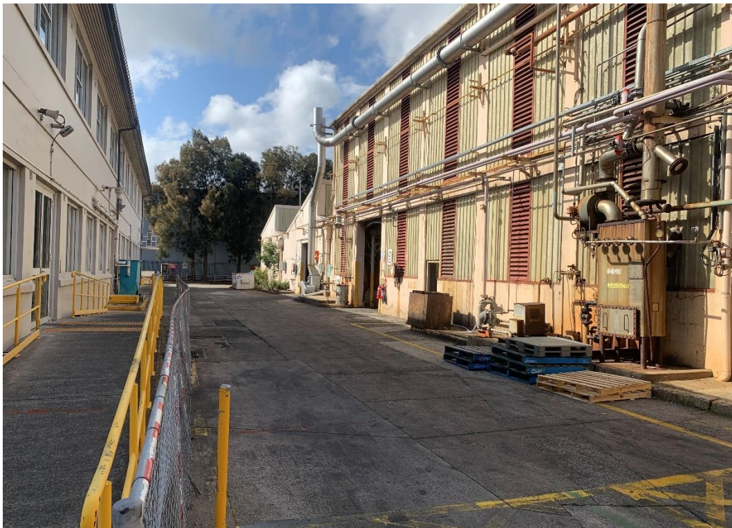
Photo 14: Looking North with Alkyd Resin Plant on Right and Administration Building on Left
