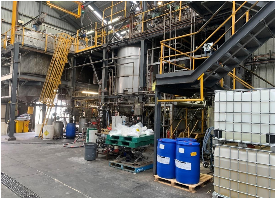
Photo 42: Emulsions Plant Building (East)
