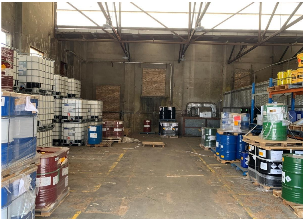
Photo 69: Poisons and Corrosive Storage Area (east)
