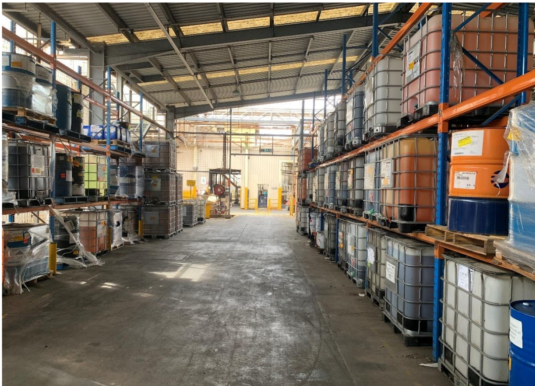
Photo 60: Drum Storage Building (West)
