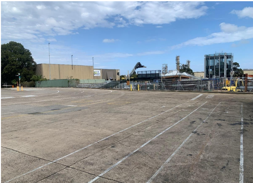
Photo 88: Truck Loading and Turning Area (Looking South-East Towards the Coal Pier Road Driveway Entrance)
