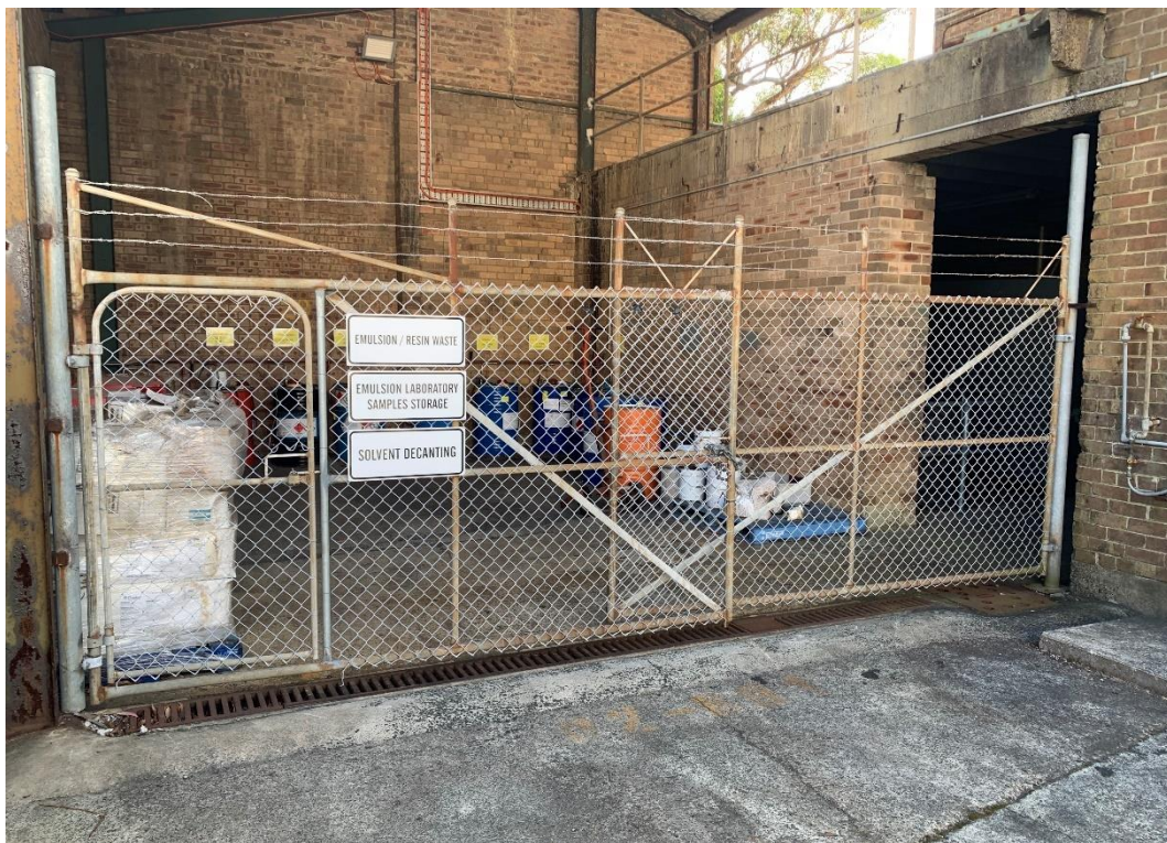
Photo 5: Waste Storage and Laboratory Sample Storage Area
