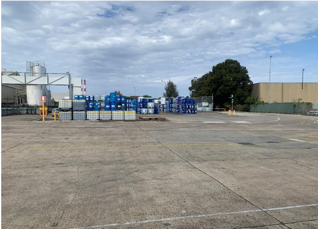
Photo 89: Truck Loading and Turning Area and External Bunded Storage Area South of Nuodex Plant (Looking East)
