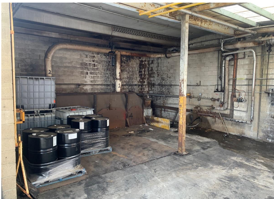
Photo 80: Undercover Storage Area South of the Hard Resin Plant
