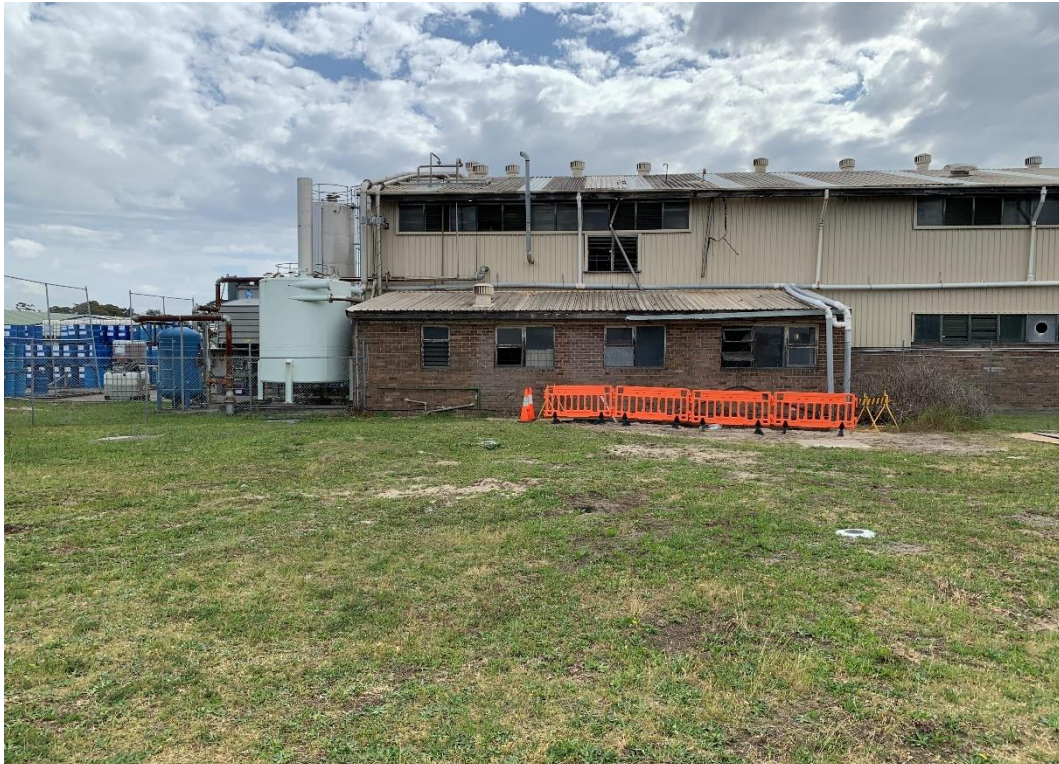
Photo 115: Nuodex Plant Spill Area Barricaded Off (Looking West)
