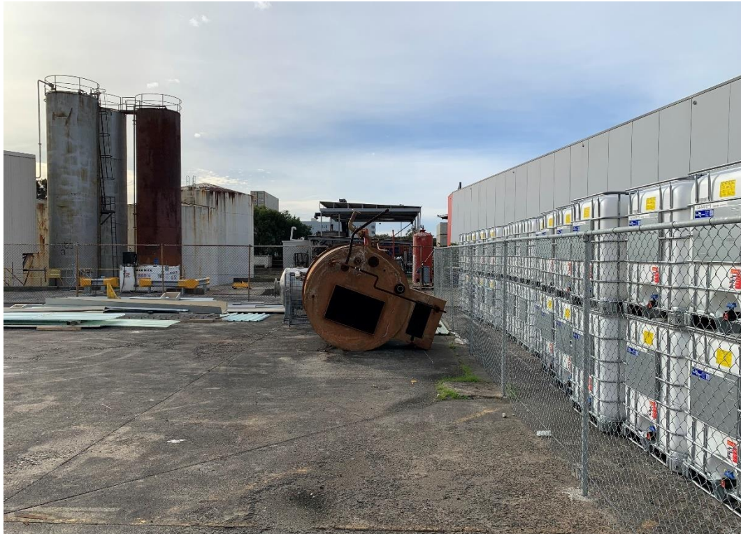
Photo 107: Eastern Staff Car Park, Storage and AST Area (Looking North)
