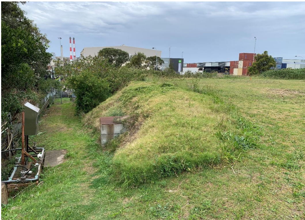
Photo 120: Eastern Grass Area and North-Eastern Site Boundary (Looking East Towards Access Gate for Stormwater Pits)
