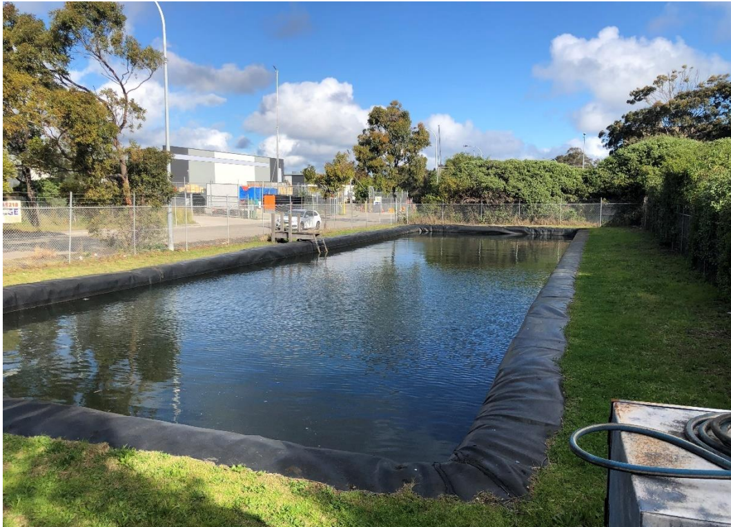
Photo 125: Stormwater First Flush Pit Overflow Basin (Looking South-East)
