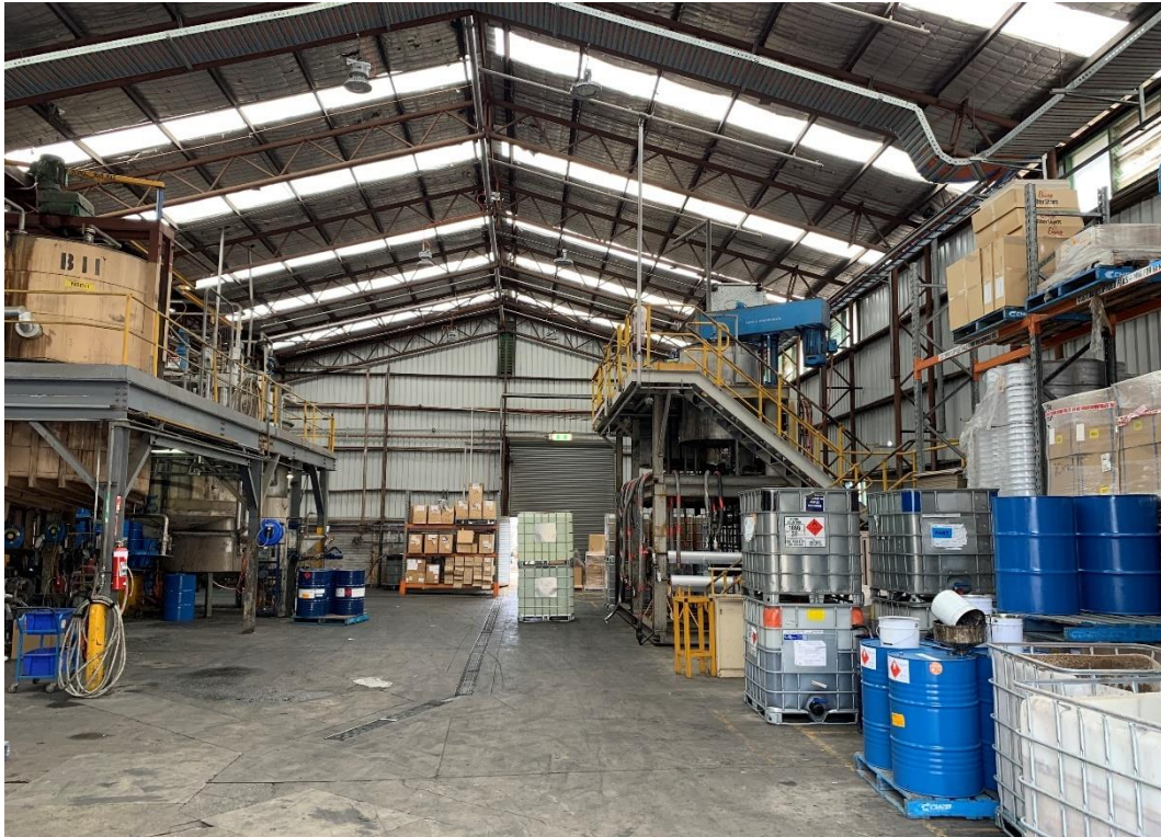
Photo 111: Nuodex Plant (West)
