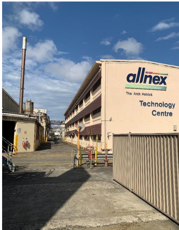
Photo 8: Looking East Through Centre of Site with Offices and Laboratories on the Right and Alkyd Plant on the Left
