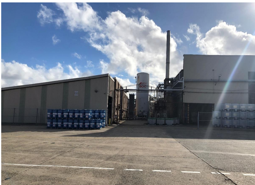
Photo 82: Hard Resin Plant, Liquid Nitrogen AST, Corrosives Storage Room and Truck Loading Area (Looking West)
