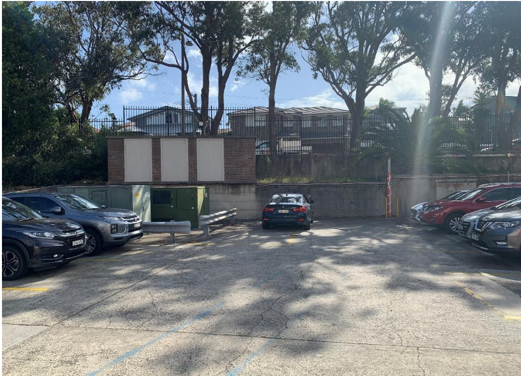
Photo 9: Western Staff Car Park (Looking West Towards Substations and Stephen Road)
