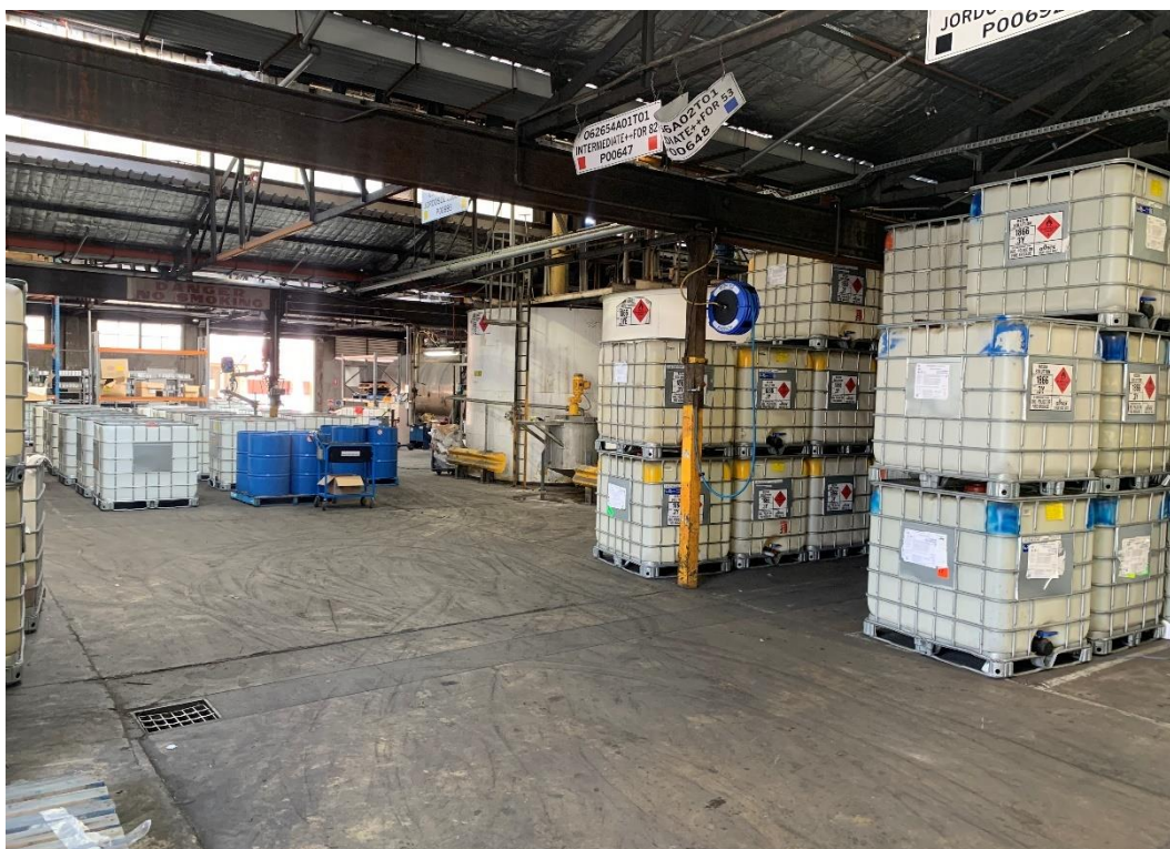
Photo 21: Alkyd Resin Plant Production and Storage Area (Looking Sout-West)
