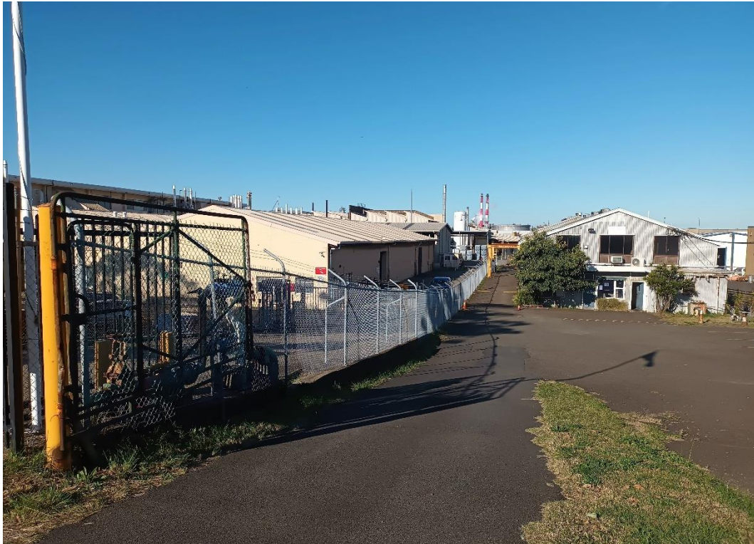
Photo 129: Adjacent Industrial Property to the South (Looking East from Stephen Road)
