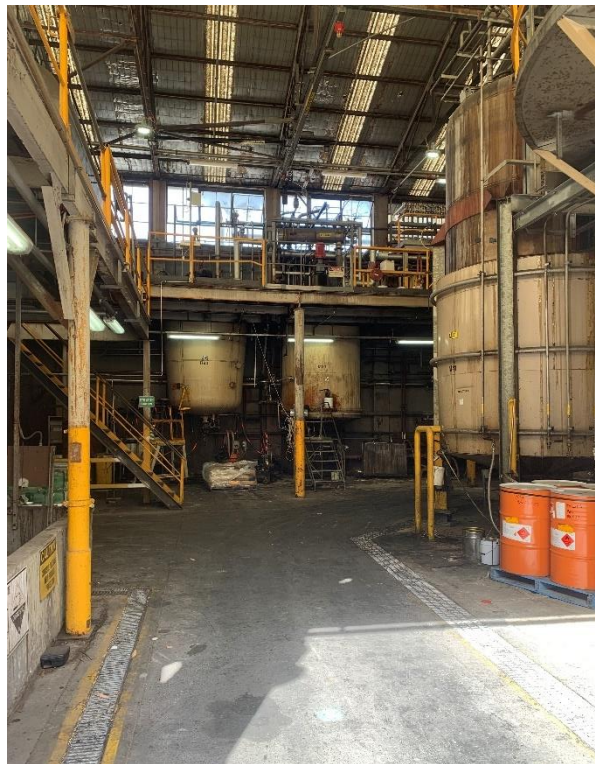
Photo 18: Alkyd Resin Plant Thinning Room
