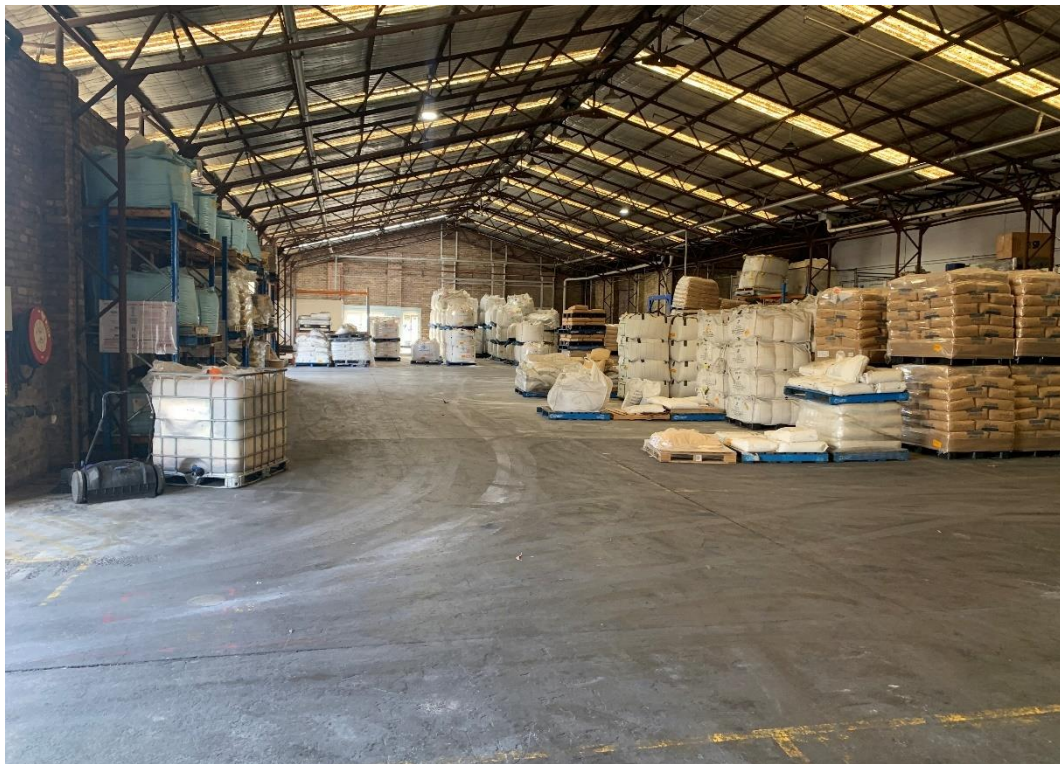
Photo 28: Raw Storage Building (Looking West)
