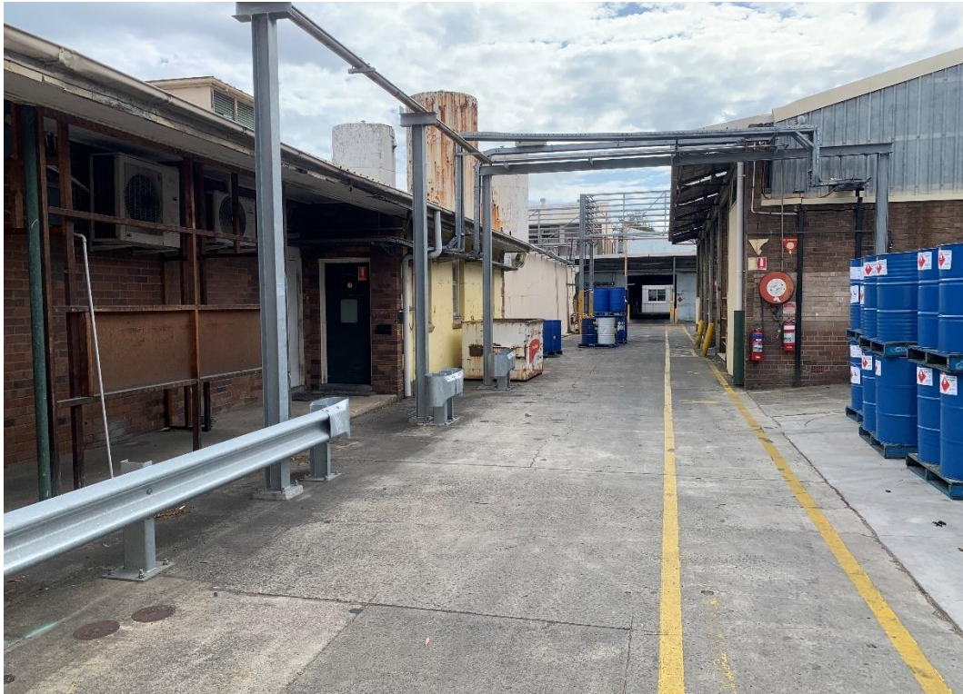
Photo 39: Emulsions Plant Control Room Building and Northern UST Farm Pump Room
