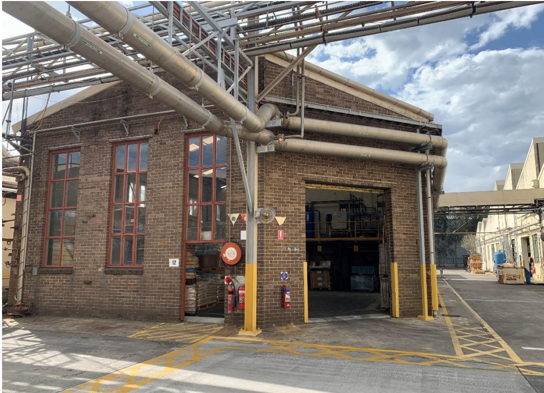
Photo 55: Brick Building - Storage and Water Plant Room
