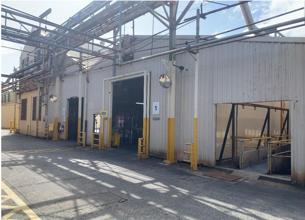
Photo 49: Beckamine Plant (Looking North-West)
