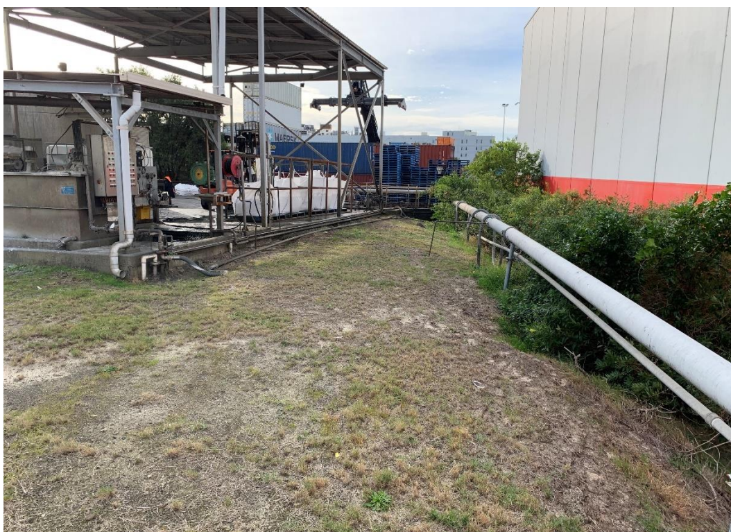
Photo 100: North-Eastern Corner of Site and Wastewater Treatment Plant
