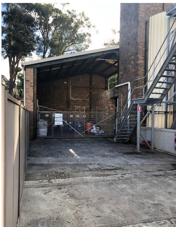
Photo 6: Former Substation Area
