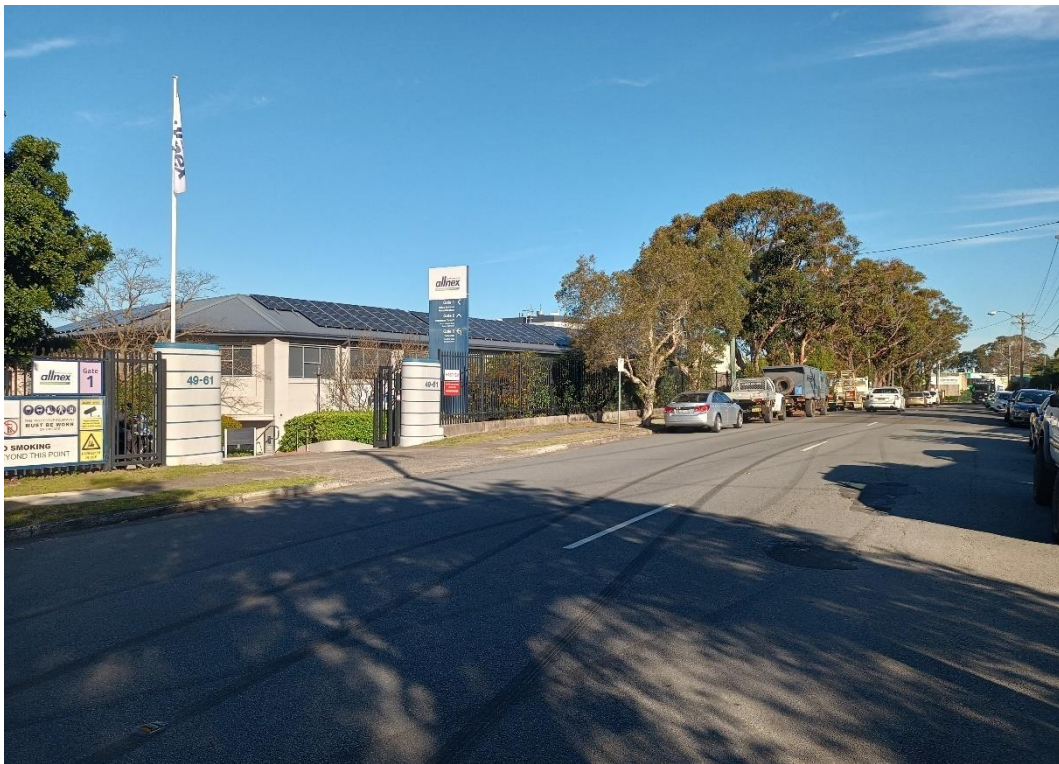
Photo 132: Main Site Entrance Off Stephen Road
