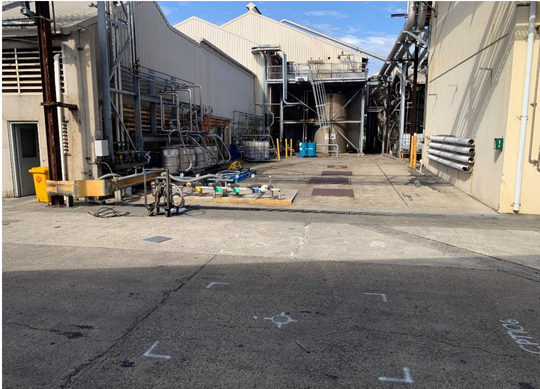
Photo 47: Central UST Farm Between Emulsions and Beckamine Plants (Looking East)
