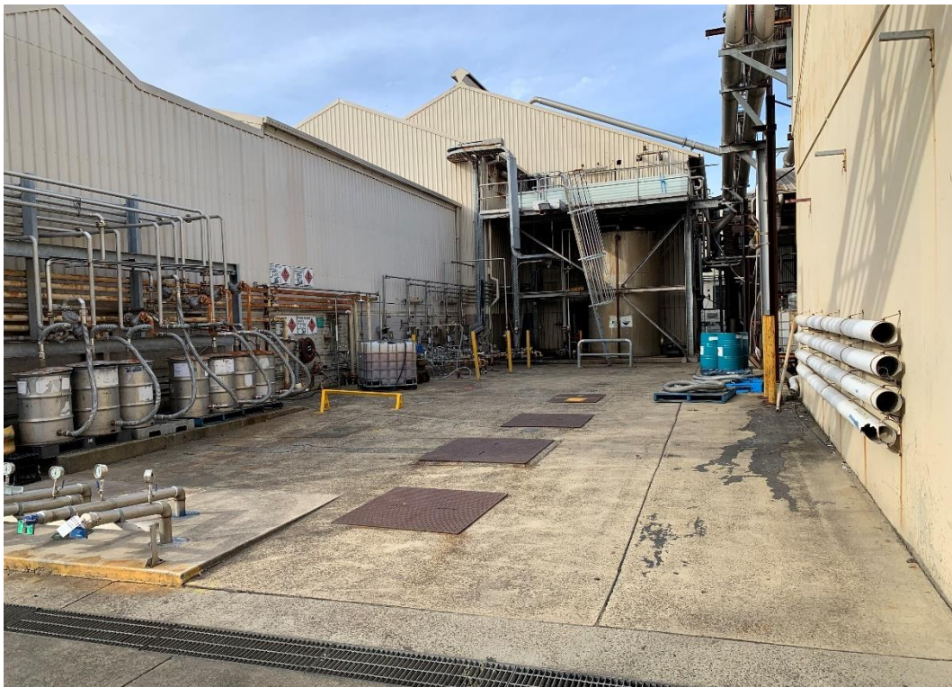
Photo 48: Central UST Farm Between Emulsions and Beckamine Plants (Looking East)
