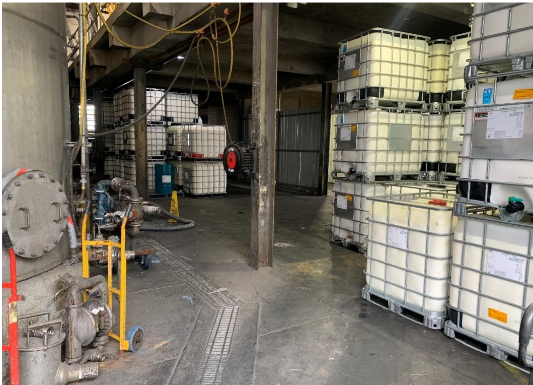
Photo 74: Southern End of Emulsions Plant Storage Building - AST and IBCs
