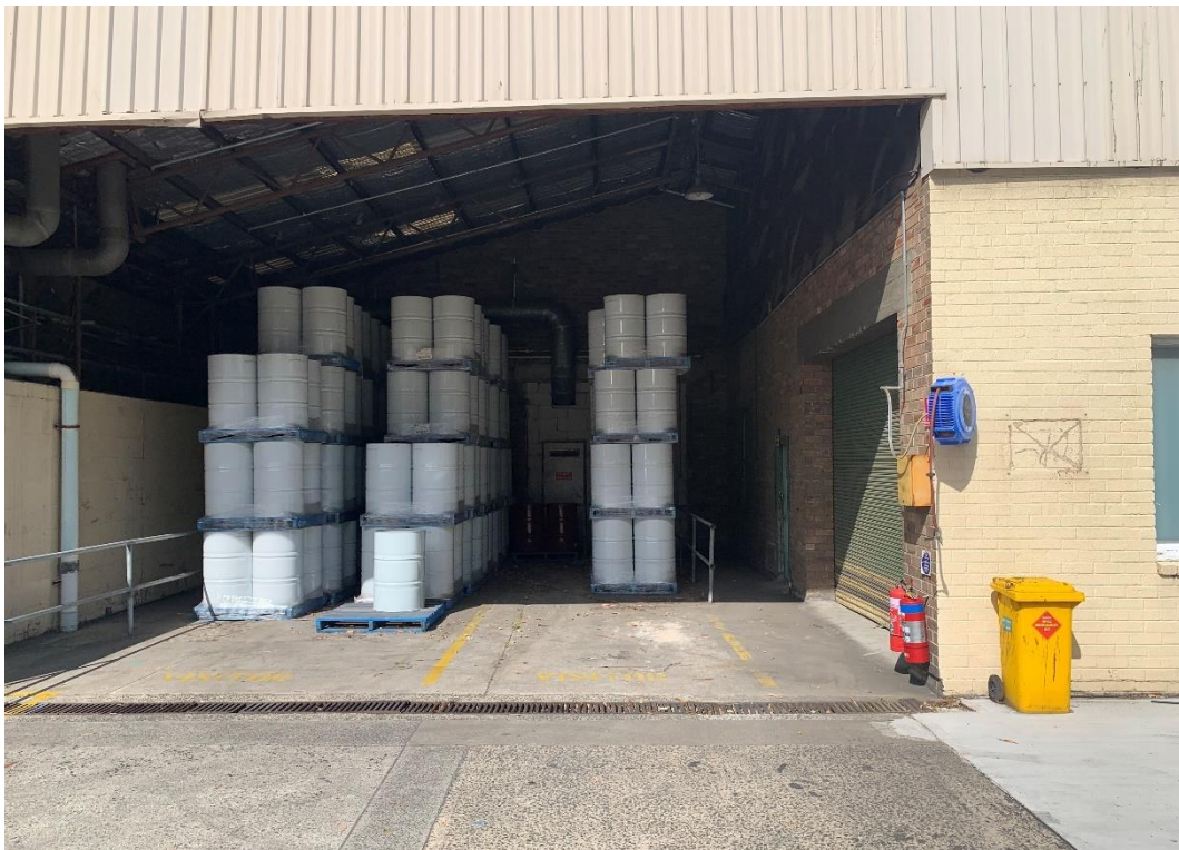
Photo 26: Loading Dock at Western End of Laboratory and Raw Materials Storage Building
