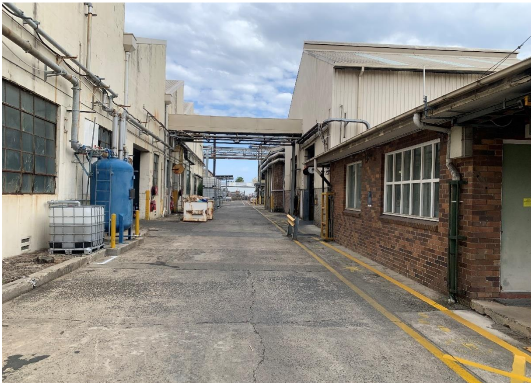
Photo 44: Between Emulsions Plant and Storage Buildings (Looking South)
