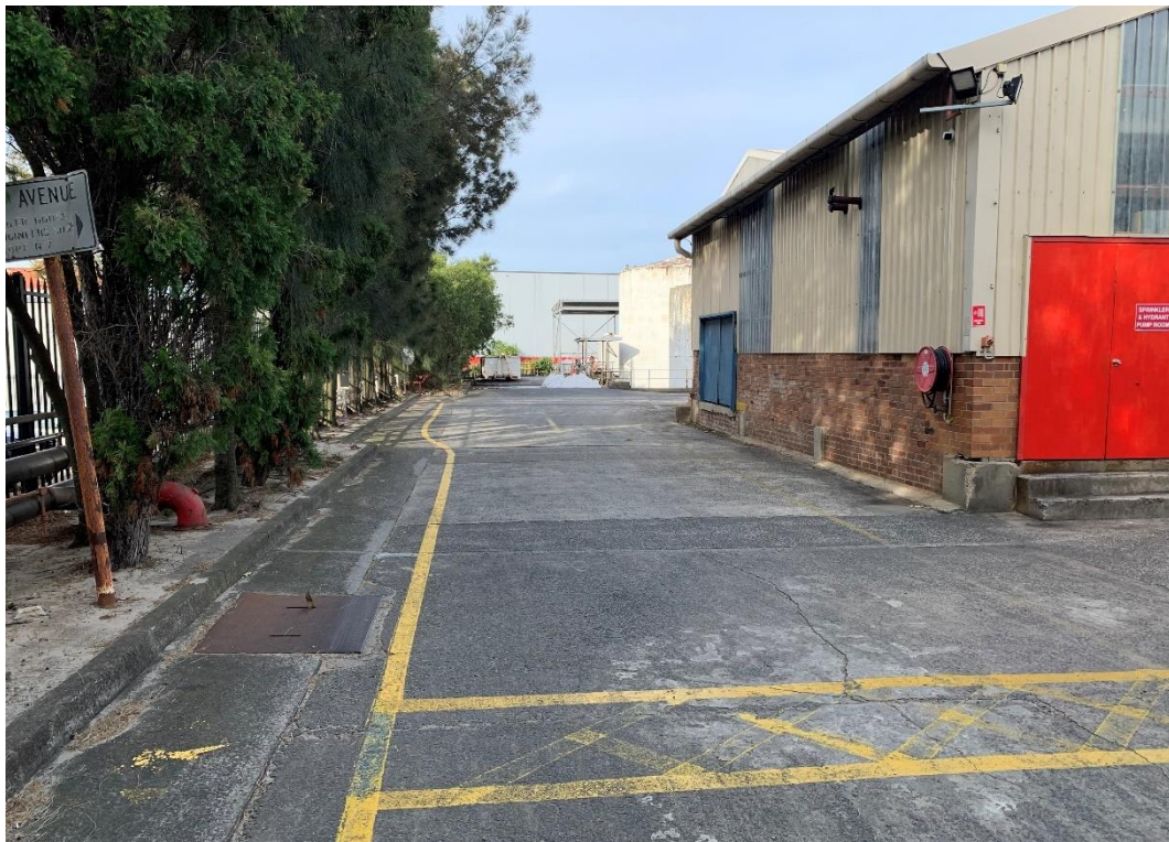
Photo 94: Fire Sprinkler and Hydrant Pump Room (Looking East Along Northern Boundary)
