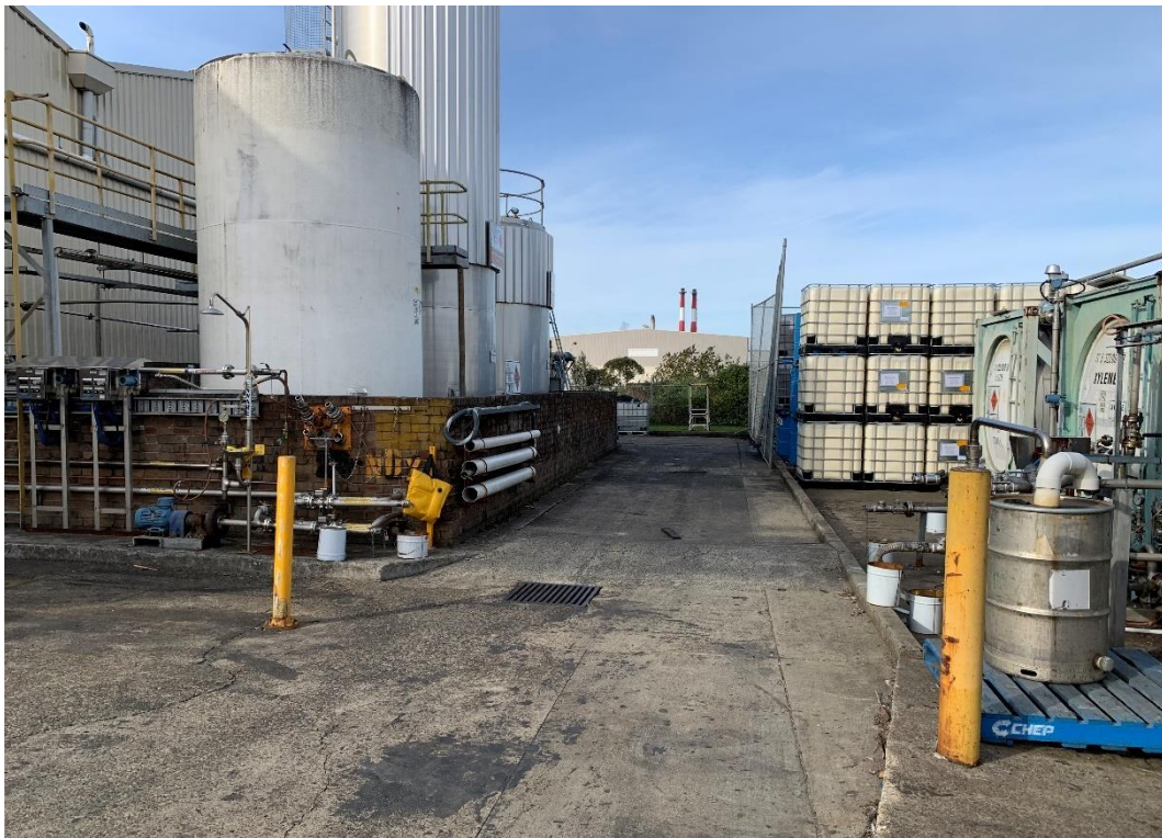
Photo 112: South-Eastes (Nuodex Plant) AST Farm (Looking East)
