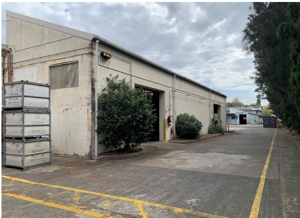
Photo 67: Northern End of Emulsions Plant Storage Building (Looking South-West)
