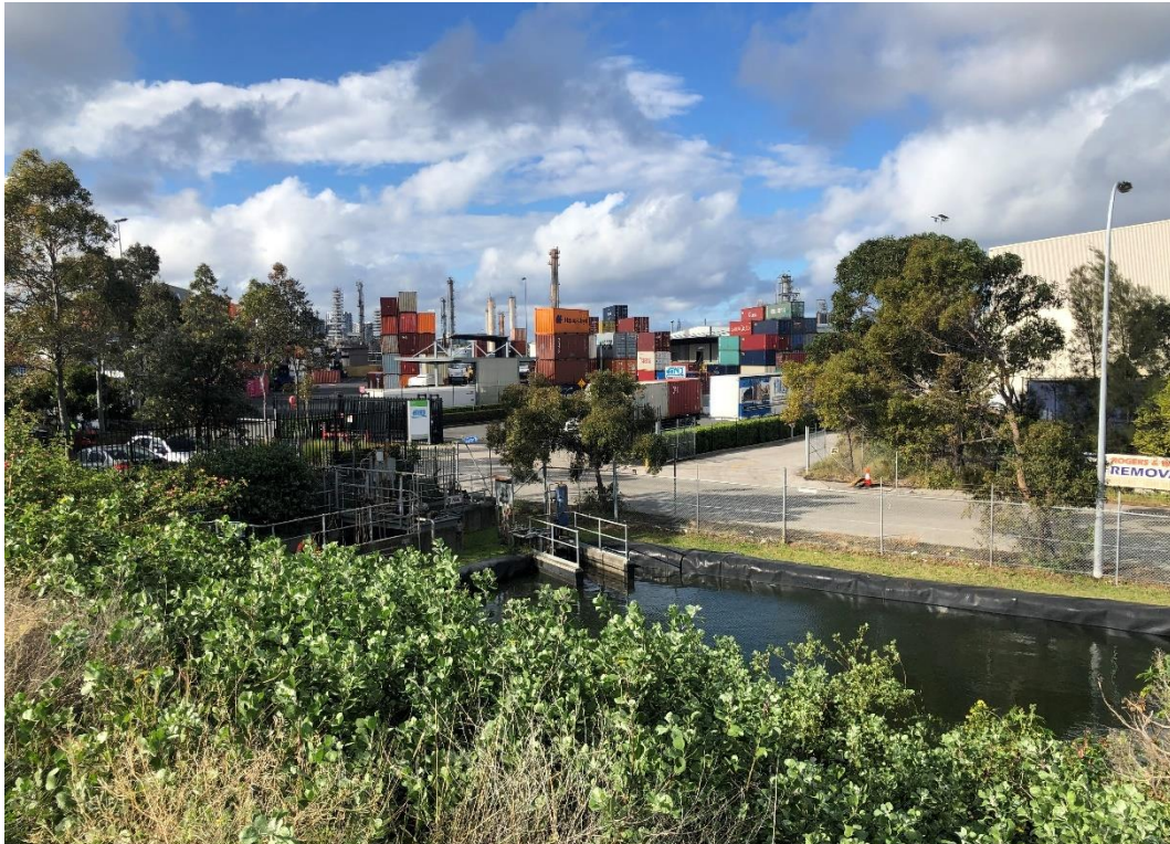
Photo 127: Adjacent Industrial Properties to the East (Looking North-East Towards Coal Pier Road)
