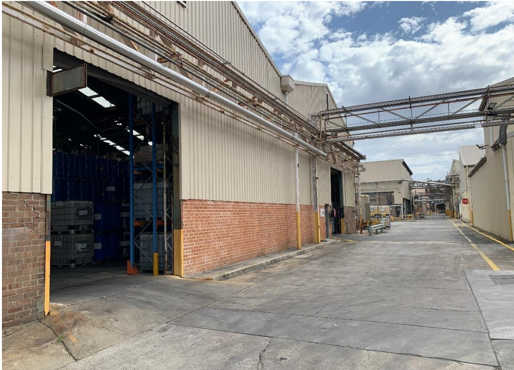
Photo 109: Looking West Through Centre of the Site from the Nuodex Plant
