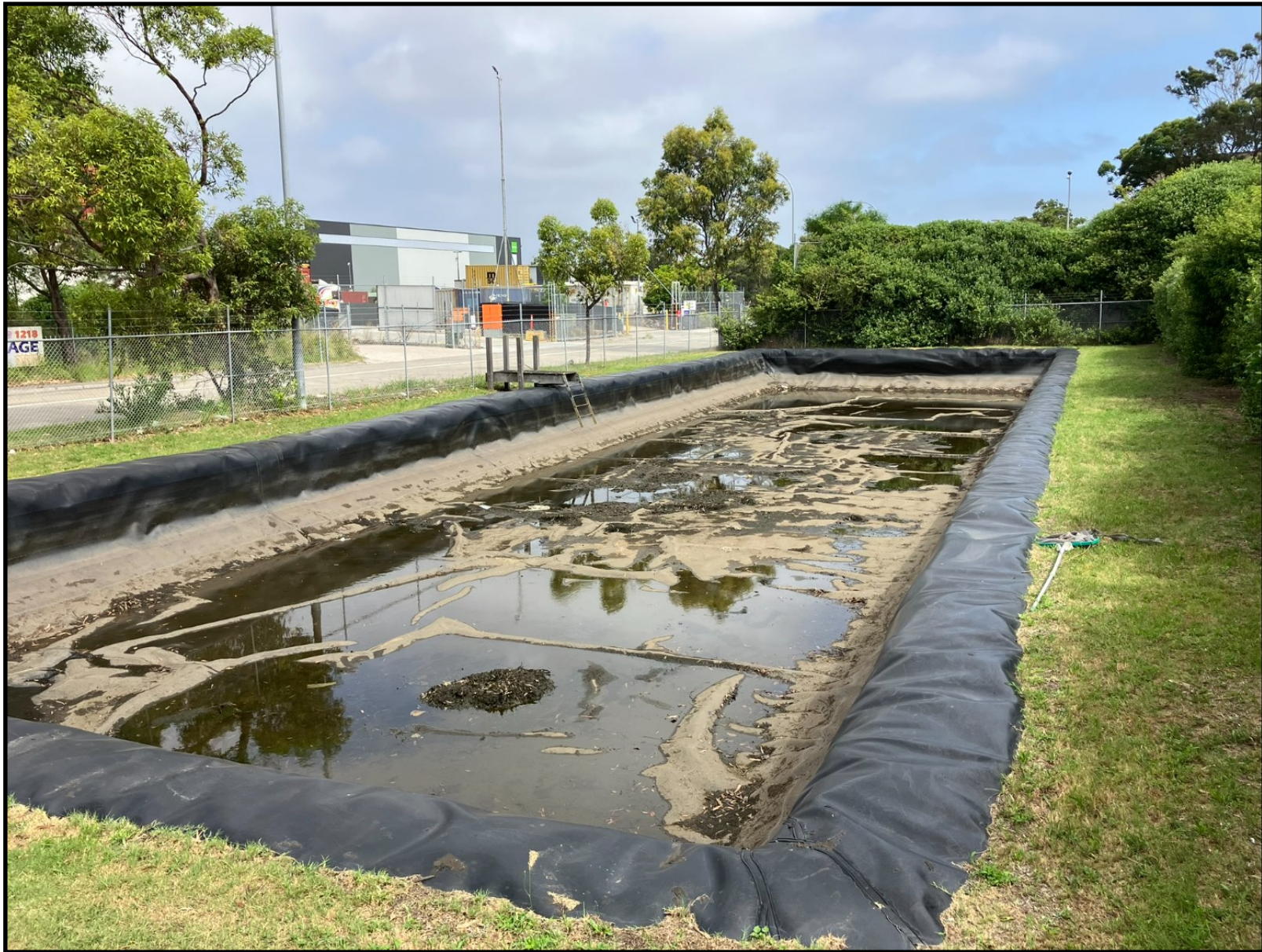
Photograph 8: Existing stormwater detention ponds occurring on-site
