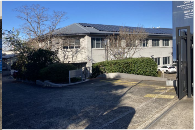
Photo 4.12 Administration building, showing the west elevation.
