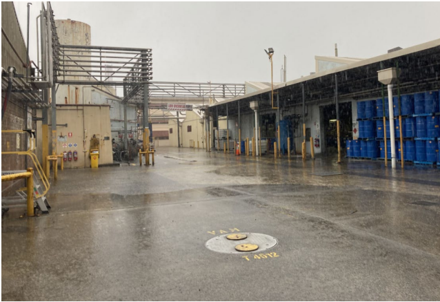
Photo 4.11 Centre of the Project Area, showing lid and marker of one of the underground tanks.
