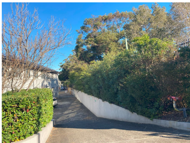
Photo 4.3 Retaining wall along west boundary showing variation in level between the street and Project Area.
