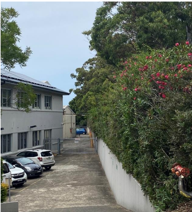
Picture 3 Retaining Wall Along Stephen Road Boundary
