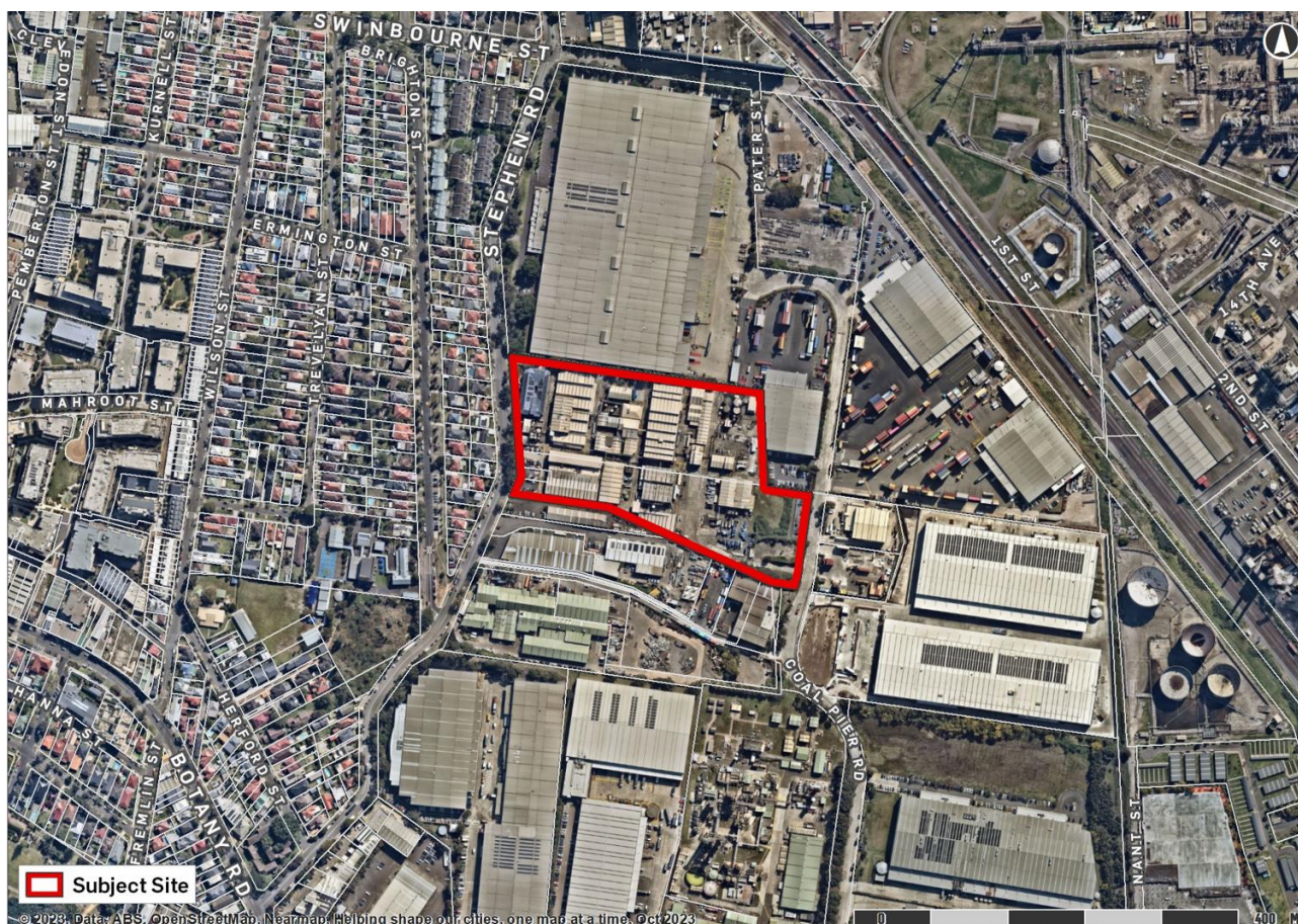
Figure 1 Aerial Image of Site
