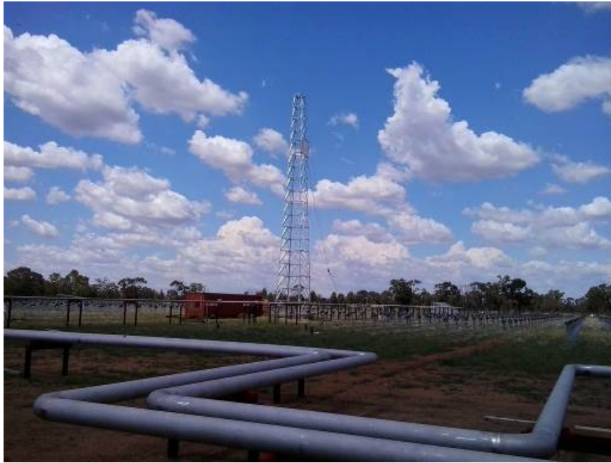
Figure 2-7 Piping prior to being insulated during construction at Pilot Plant
