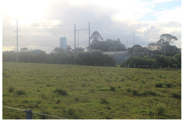
View of the neighbouring Substation to the West
