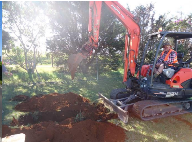
Figure 5: North facing in the location of test pit TP 12.
