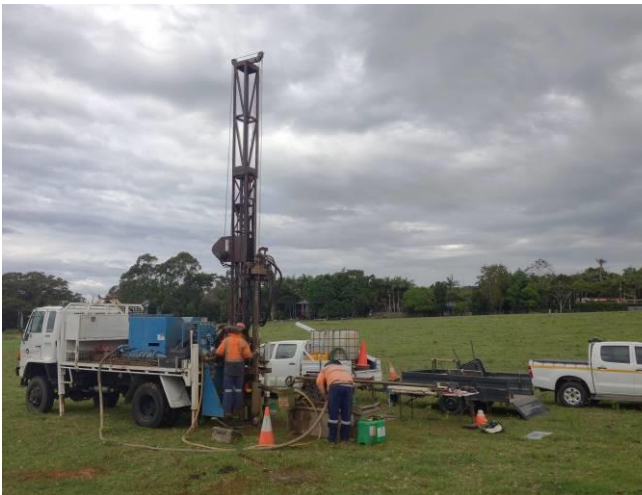
Figure 2: South-east facing in the location of BH 2
