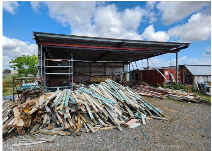
Figure 8 Shed in northern portion of the site
