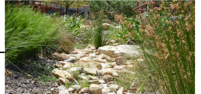
Loose rock bed swale with WSUD sensitive planting
