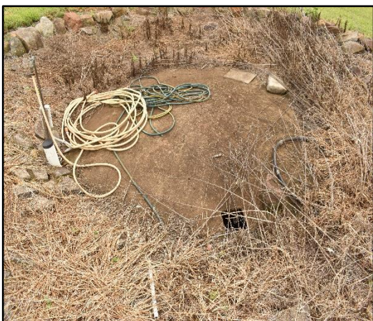
Figure 37: Detail of small extant concrete cistern
