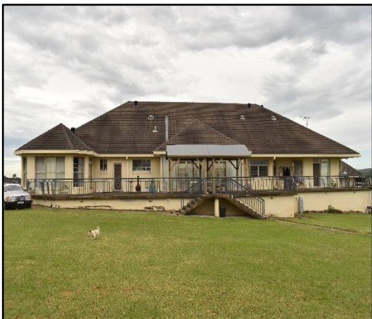
Figure 25: Large residential building, view south
