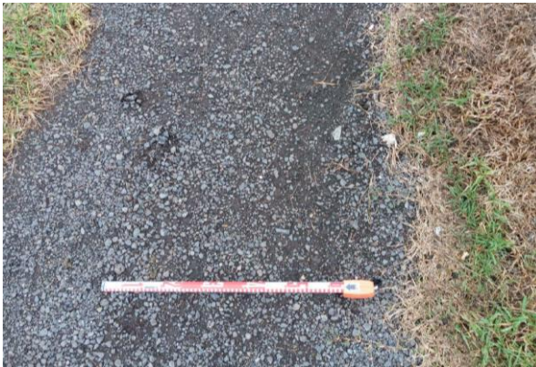
Figure 17: Unsealed driveway. Imported blue metal fill
