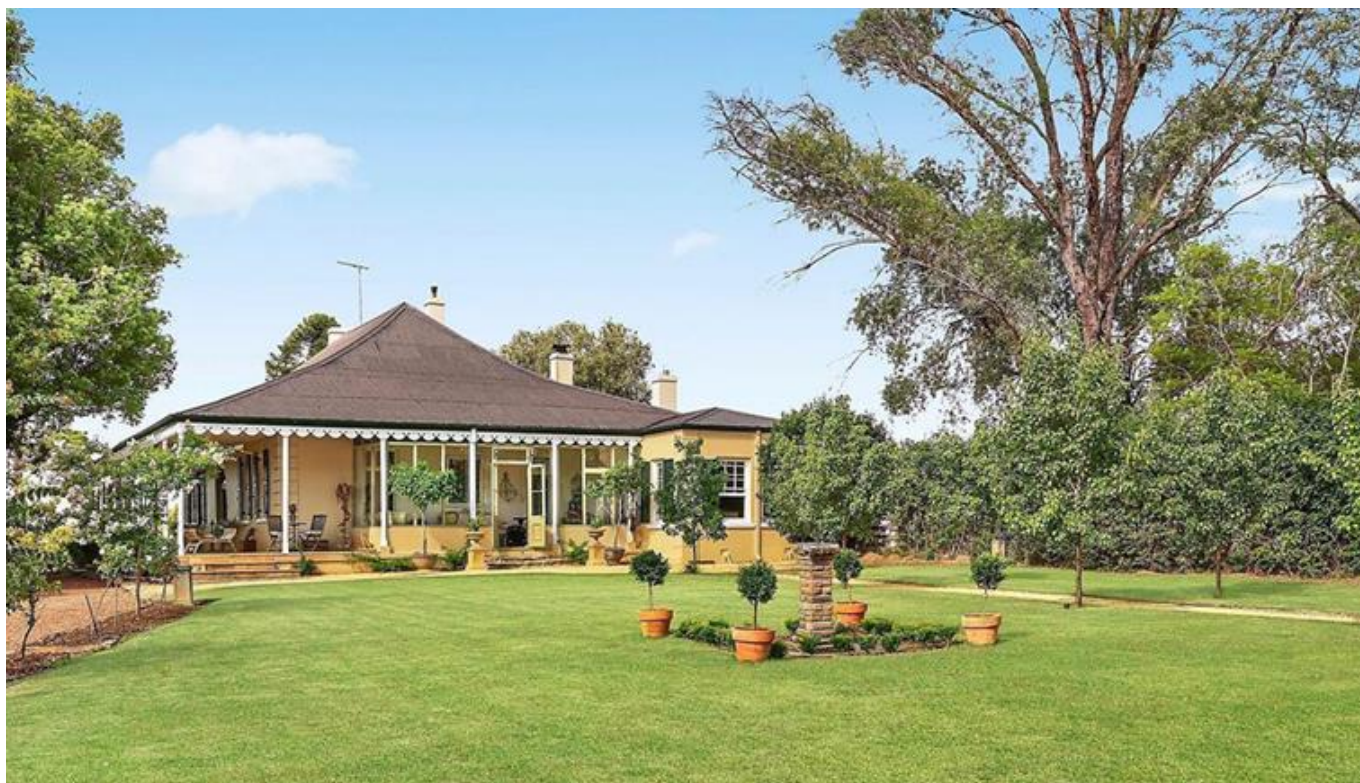
Figure 7 Kelvin Park Homestead main homestead structure
