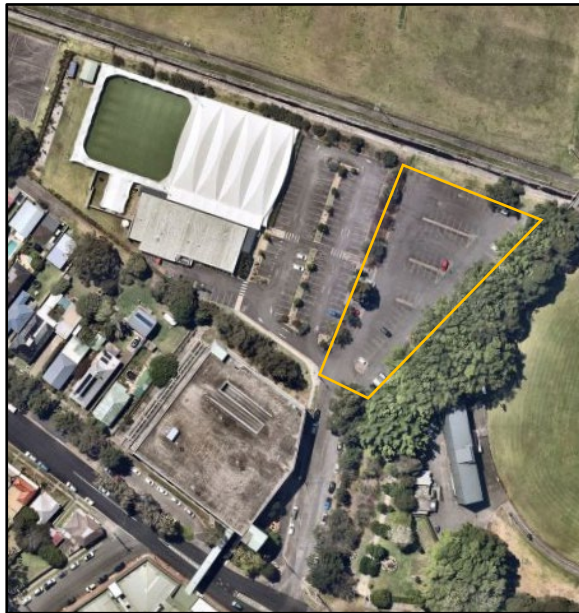
Figure 2-9 Off-street parking adjacent to Harker Oval Stadium
