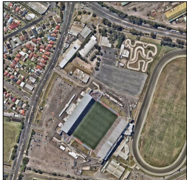
Figure 2-10 Off-street parking surrounding McDonald Jones Stadium
