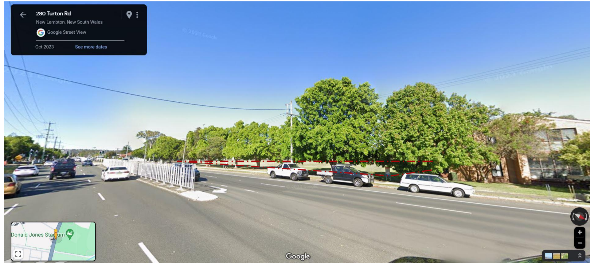
PHOTO 1 - TURTON RD - FACING SOUTH-WEST
