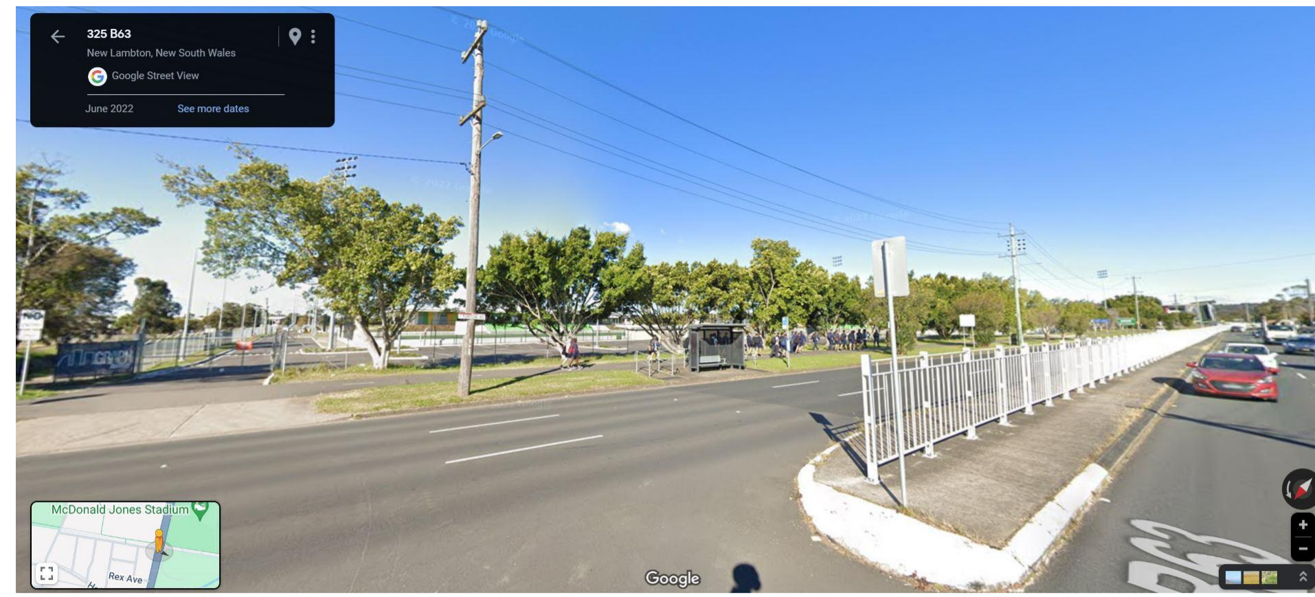
PHOTO 8 - CNR. TURTON & MONASH RDs - FACING SOUTH-EAST
