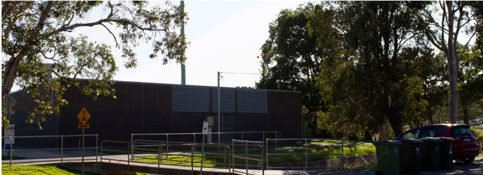
Image 49 Viewpoint 3, one frame, existing view. NOTE: The balloon is not applicable, as the proposal has been setback an additional 19.5m from Turton Road since the previous SSDA submission.
