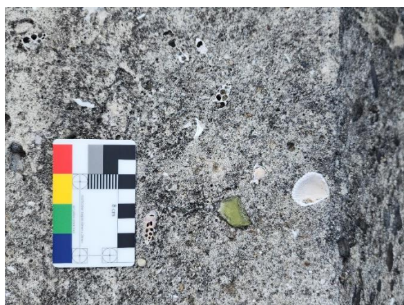
Figure 26. Detail view of stormwater channel wall showing shell and glass embedded within the concrete.
