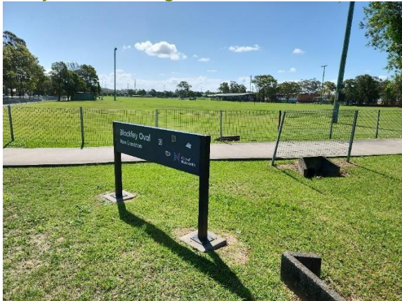
Figure 16. View west from east boundary of study area showing culverts.
