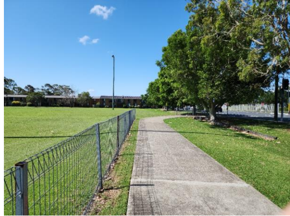
Figure 4-4. View north showing footpath, fence and drainage area under the trees.
