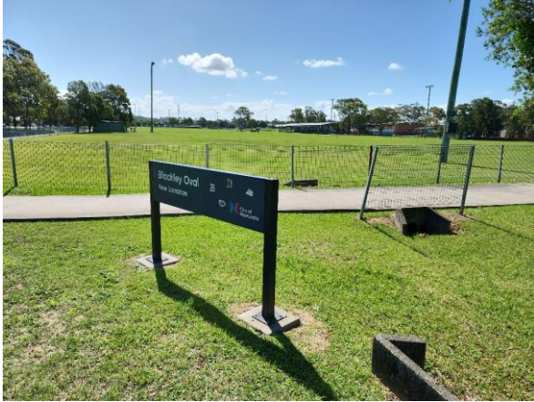
Figure 4-3. View west from east boundary of study area showing culverts.
