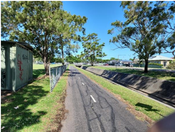
Figure 4-5. View east showing fenced edge of study area, with concrete pathway, easement and stormwater channel.
