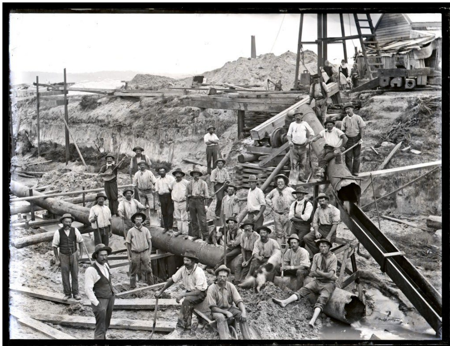
Figure 16: Drain construction workers at Broadmeadow, NSW, 6 April 1900 (Source: University of Newcastle Cultural Collections)
