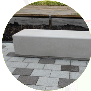
Use of green concrete to blade seating to promote reuse of site material and reduce environmental impact. Opportunity for incorporation of speakers into seating to create audible experiences of site, its history and relationships.
