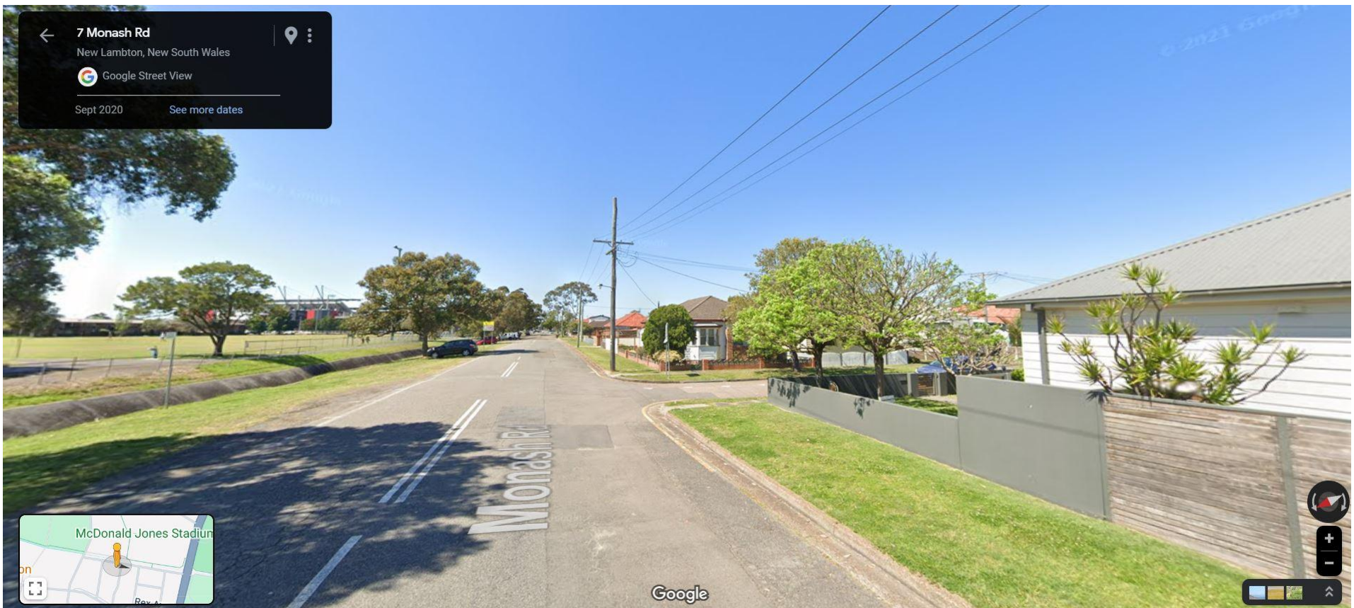
PHOTO 14 - MONASH RD - FACING EAST
