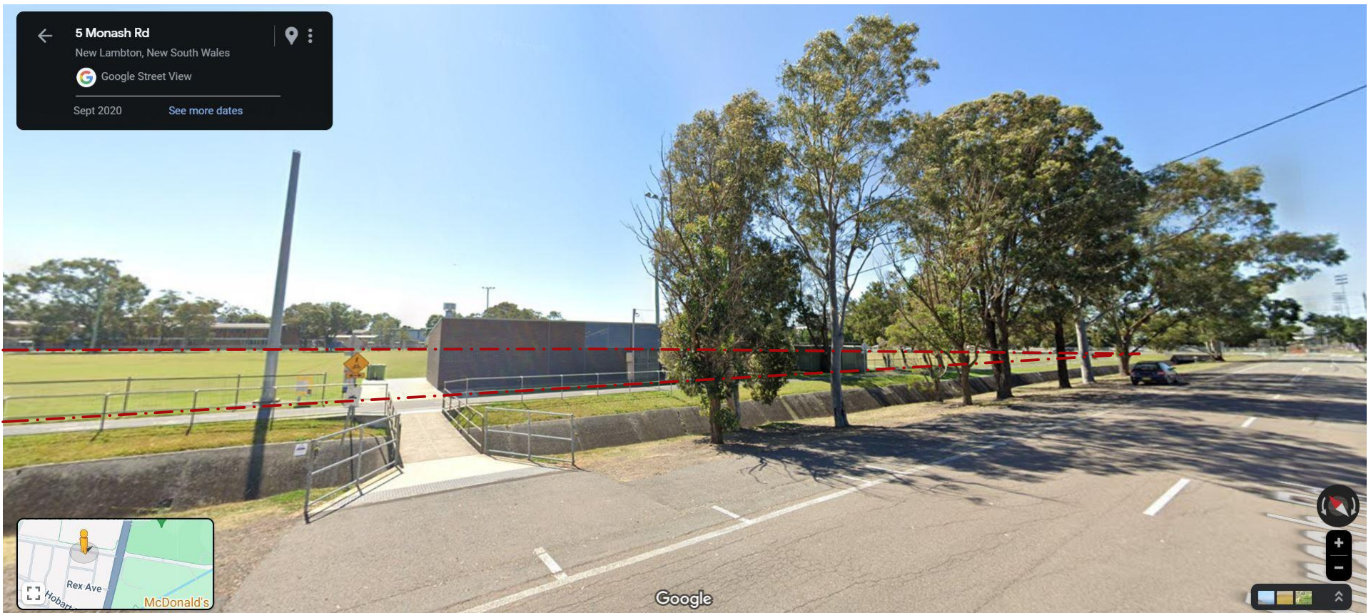
PHOTO 4 - MONASH RD - FACING NORTH-NORTH-EAST
