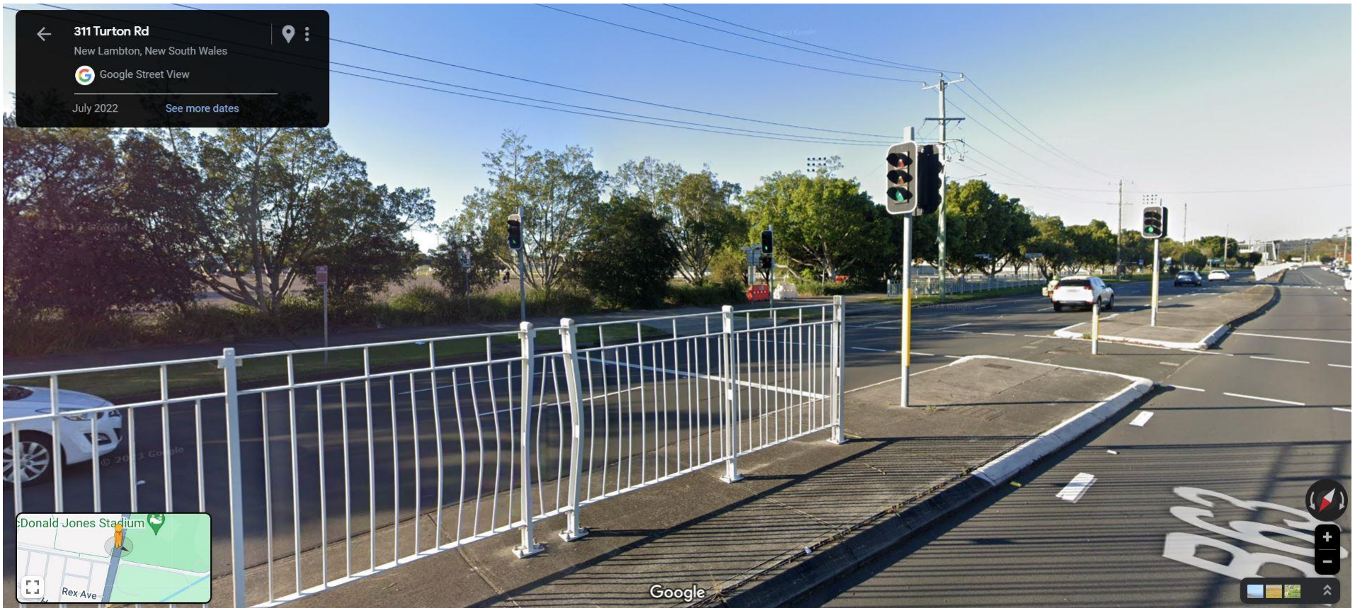
PHOTO 10 - TURTON RD - FACING SOUTH-EAST
