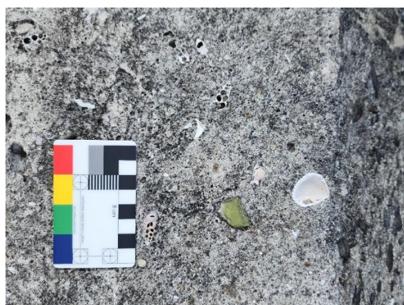
Figure 25. Detail view of stormwater channel wall showing shell and glass embedded within the concrete.
