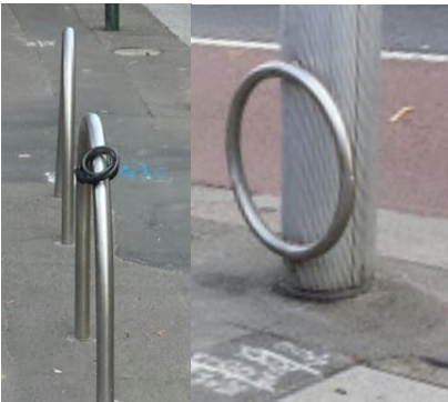
Existing U-ring & pole mounted bike racks to Broadway
