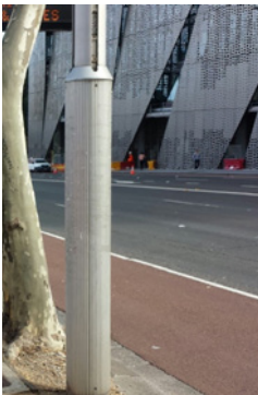
Existing Smartpole lighting to Broadway
