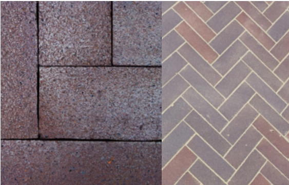
Detail brick paving in herringbone - Bowral Hamlet Blue Paver 230 x 76 x 55mm
