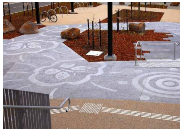
Etching on concrete footpath
