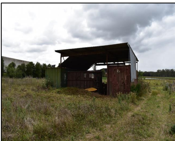
Figure 23: Detail of shed located on the northwest portion of the study area, view northeast
