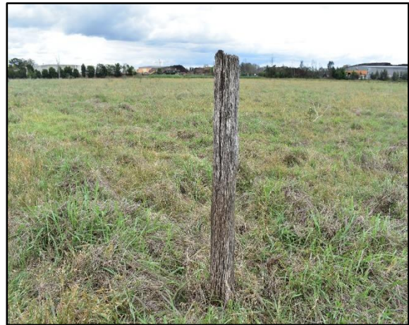
Figure 28: Detail of extant wooden fence post, view north
