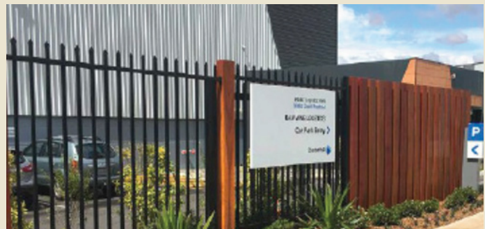
Palisade Fence with Timber Highlights
