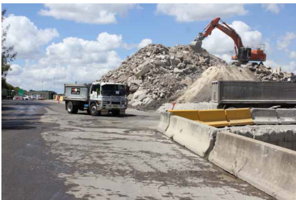
Photo 3 Incoming material stockpile
