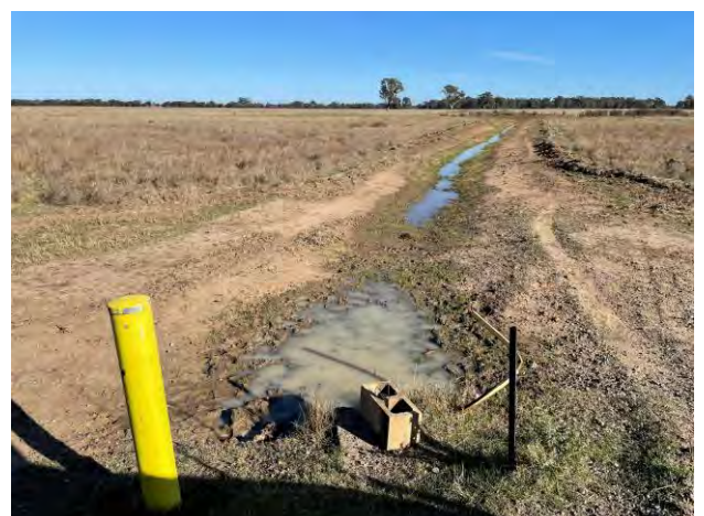
Photograph 12 - Localised surface water ponding was noted in some areas.
