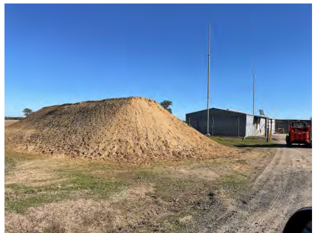
Photograph 6 - Earthen blast mounds located in the vicinity of Magazine 6.
