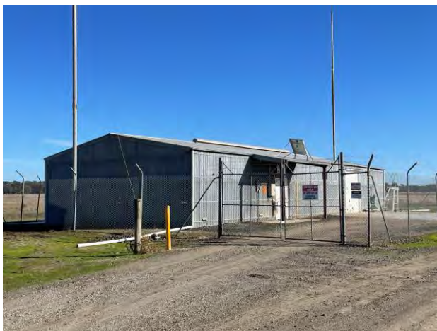
Photograph 5 - Existing magazines surrounded by security fencing.
