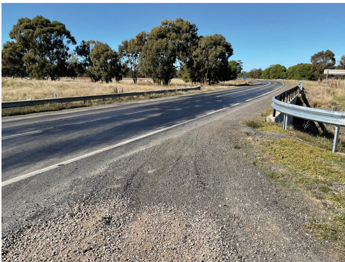
Figure 2-1 431 Newell Highway, looking south
