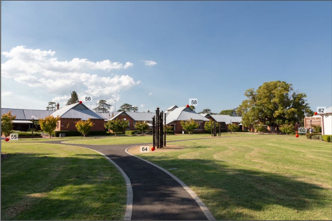
SURVEY POINTS USED FOR 3D CAMERA ALIGNMENT
