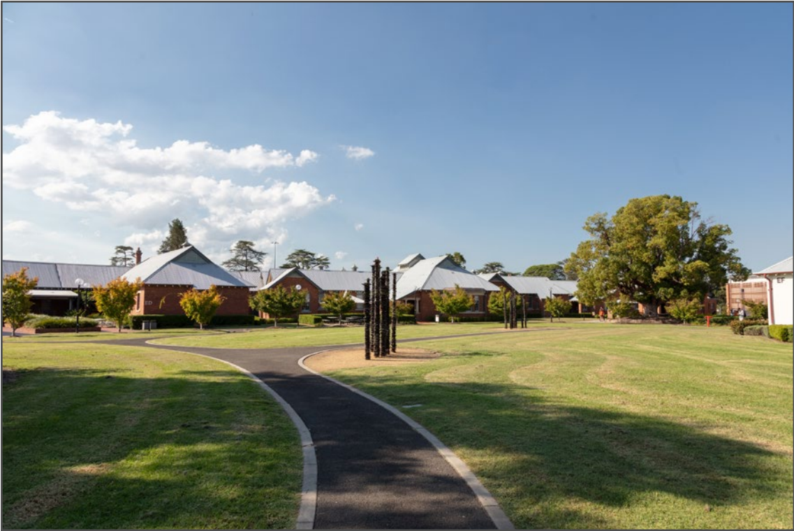
PHOTOGRAPH SHOWING EXISTING CONDITION
