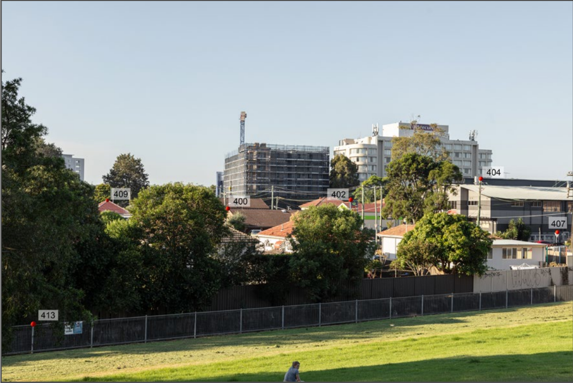
SURVEY POINTS USED FOR 3D CAMERA ALIGNMENT
