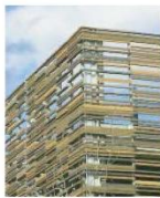
Clay Slatting • Variation of Clay Shingles • Various slats according to shading requirements
