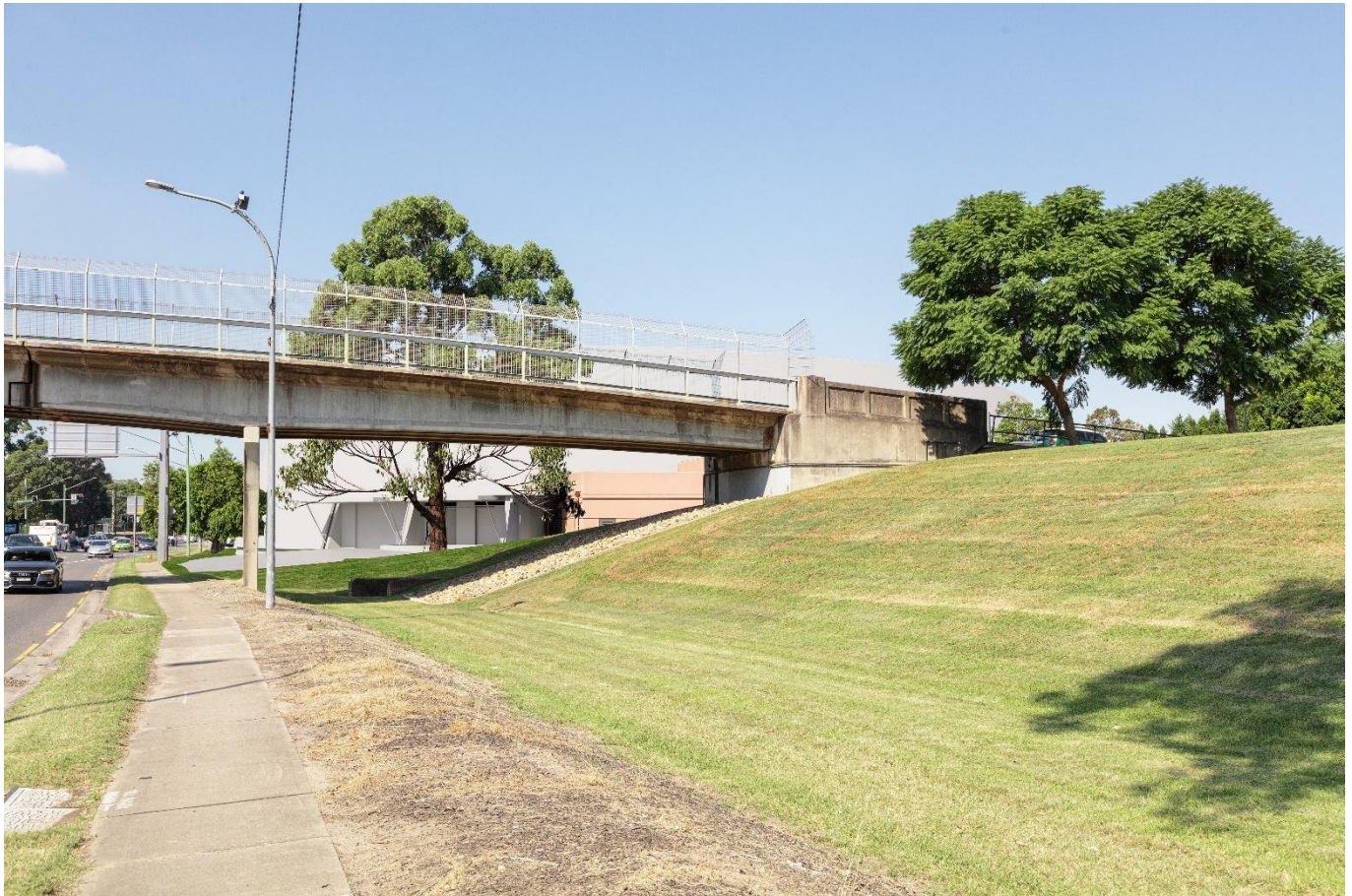
Figure 47 Visibility of the site from the north-west on the southern side of Victoria Road
