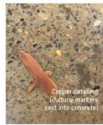
Low carbon Concrete • Theatre wall (precast) • Ground Slab (polished with exposed aggregate derived from Country)
