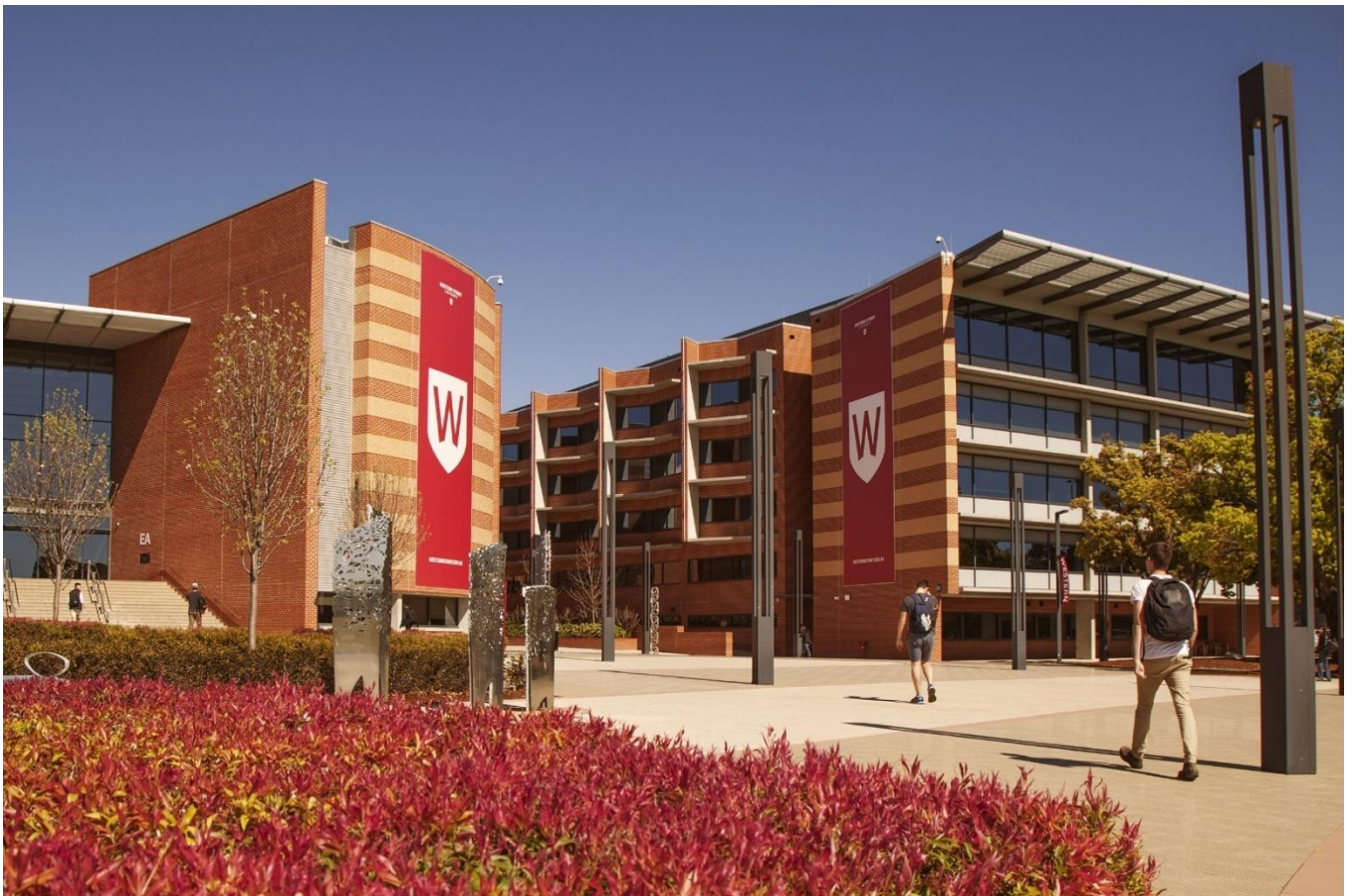
Figure 12 EA and EB buildings Source: WSU
