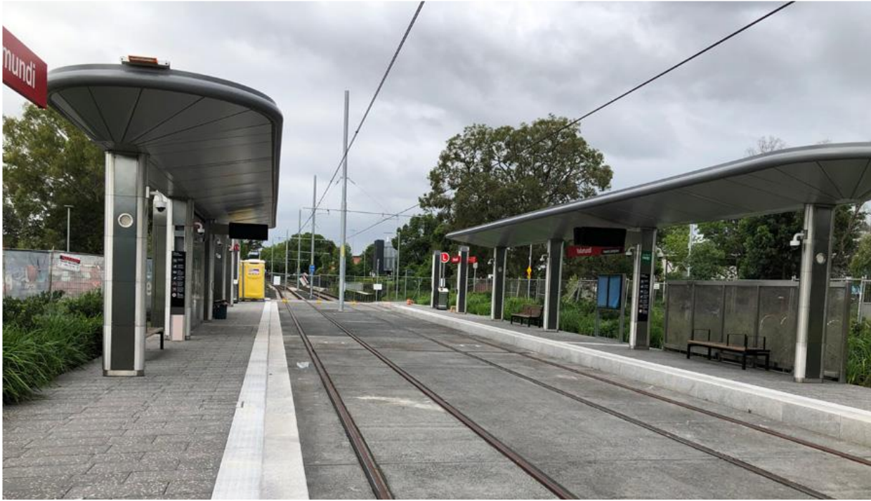
Figure 8 Yallamundi / Rydalmere Light Rail Station
