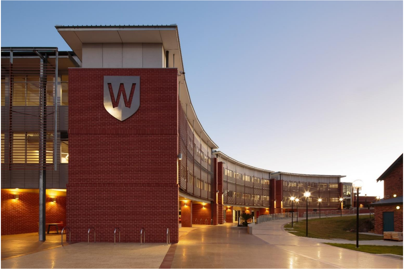
Figure 11 Eha building Source: WSU
