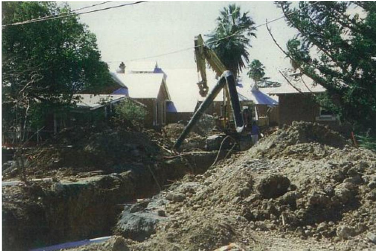
Figure 3-22: 1998 works including trenches dug for water, gas and electricity. Source: WSU 1998 pg 10 via AMBS 2024
