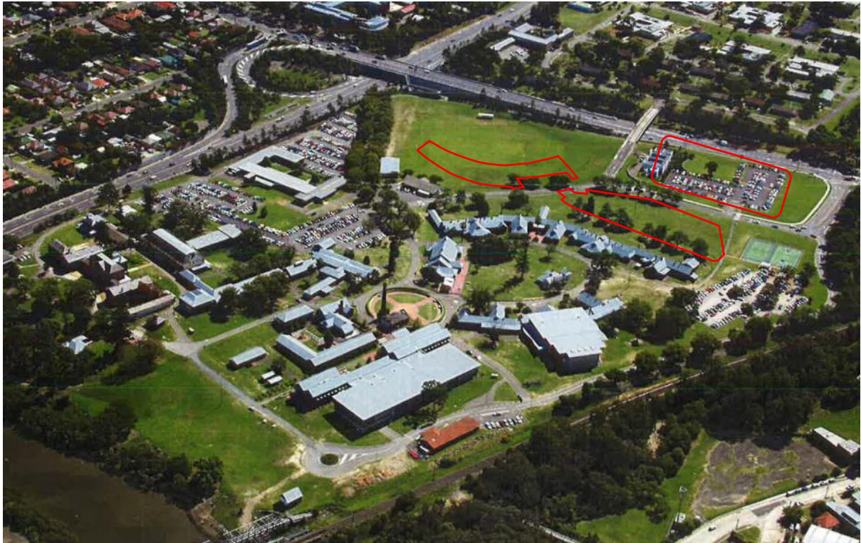
Figure 4.23: 2004 oblique aerial photograph showing the completed carpark, the Co-Generation Plant Building (Eda), grassed areas and small number of trees. The general location of the study area is shown highlighted in yellow. Source: Conybeare Morrison, 2008
