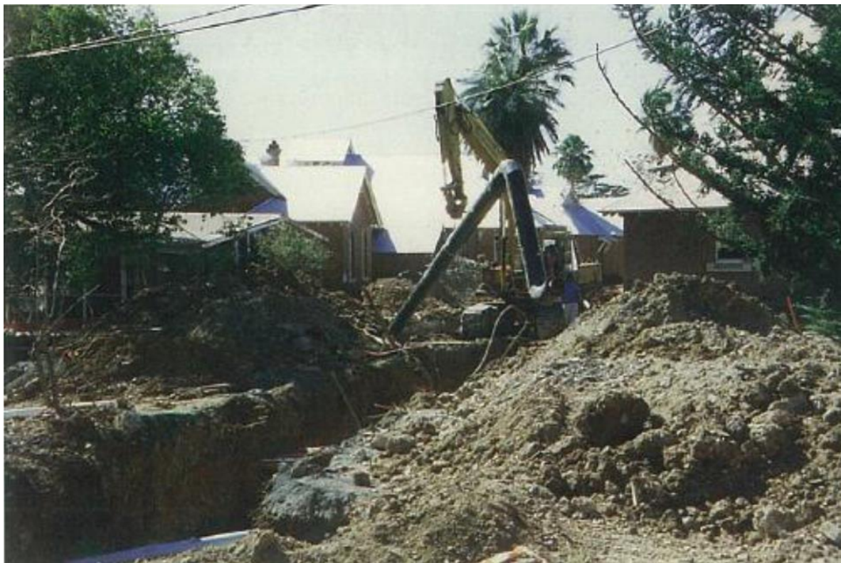
Figure 4.22: 1998 works including trenches dug for water, gas and electricity Source: WSU 1998 pg 10 via AMBS 2024
