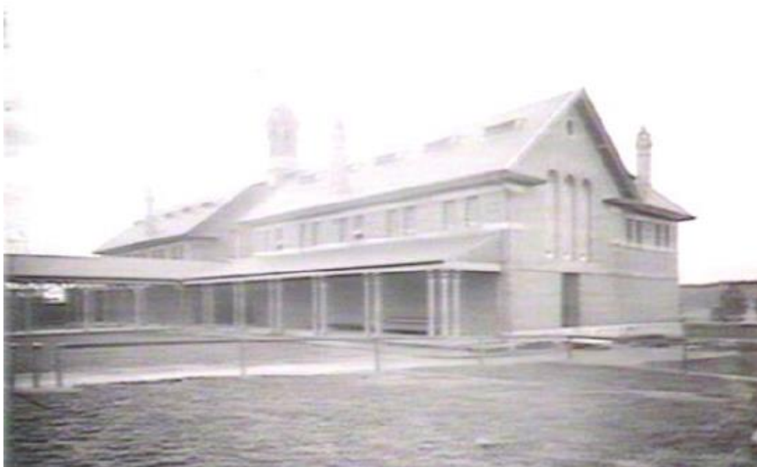
Figure 4.6: Protestant Orphan School building and covered way from central Female Orphan School building c.1870-80 Source: State Library NSW, Government Printing Office 1 - 06149
