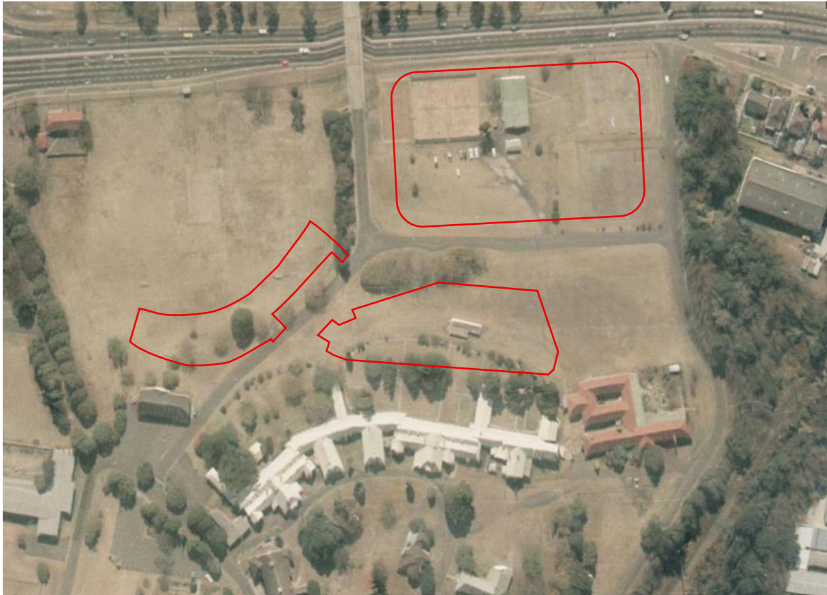
Figure 4.20: 1986 aerial photograph showing the addition of shade structures along the northern and southern sides of the tennis courts, the use of the area to the south of the courts for parking and an informal driveway between the southern boundary and the tennis courts. Source: Historical Imagery NSW
