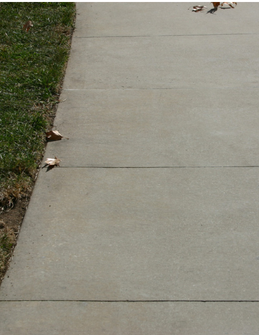
in situ concrete paving
