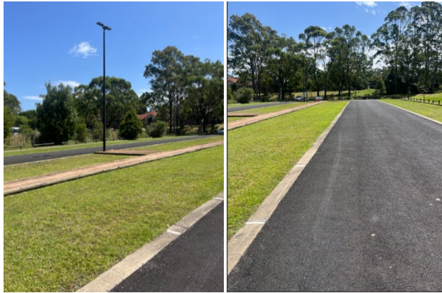
Figure 4 Photos of the Turf-Cell Carpark at Macquarie University.
