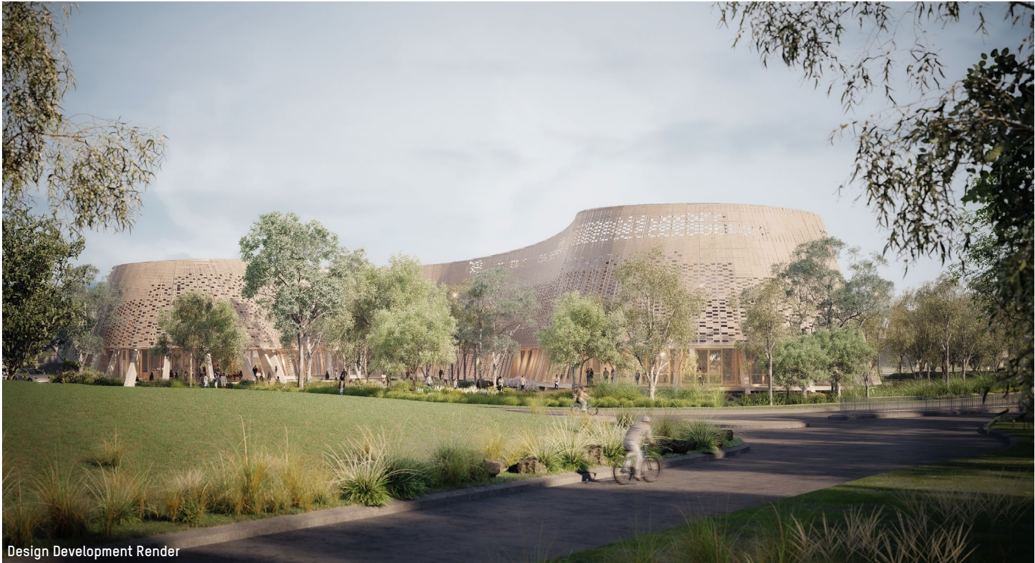
VIEW 02: Railway street & Fifth Street Round about
