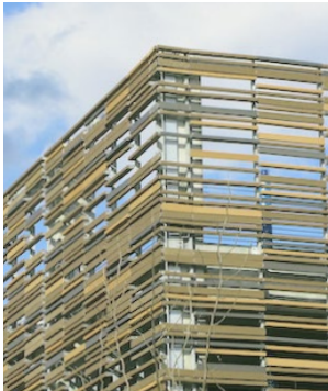
Clay Battens • Variation of Clay Shingles • Various sizes according to shading requirements
