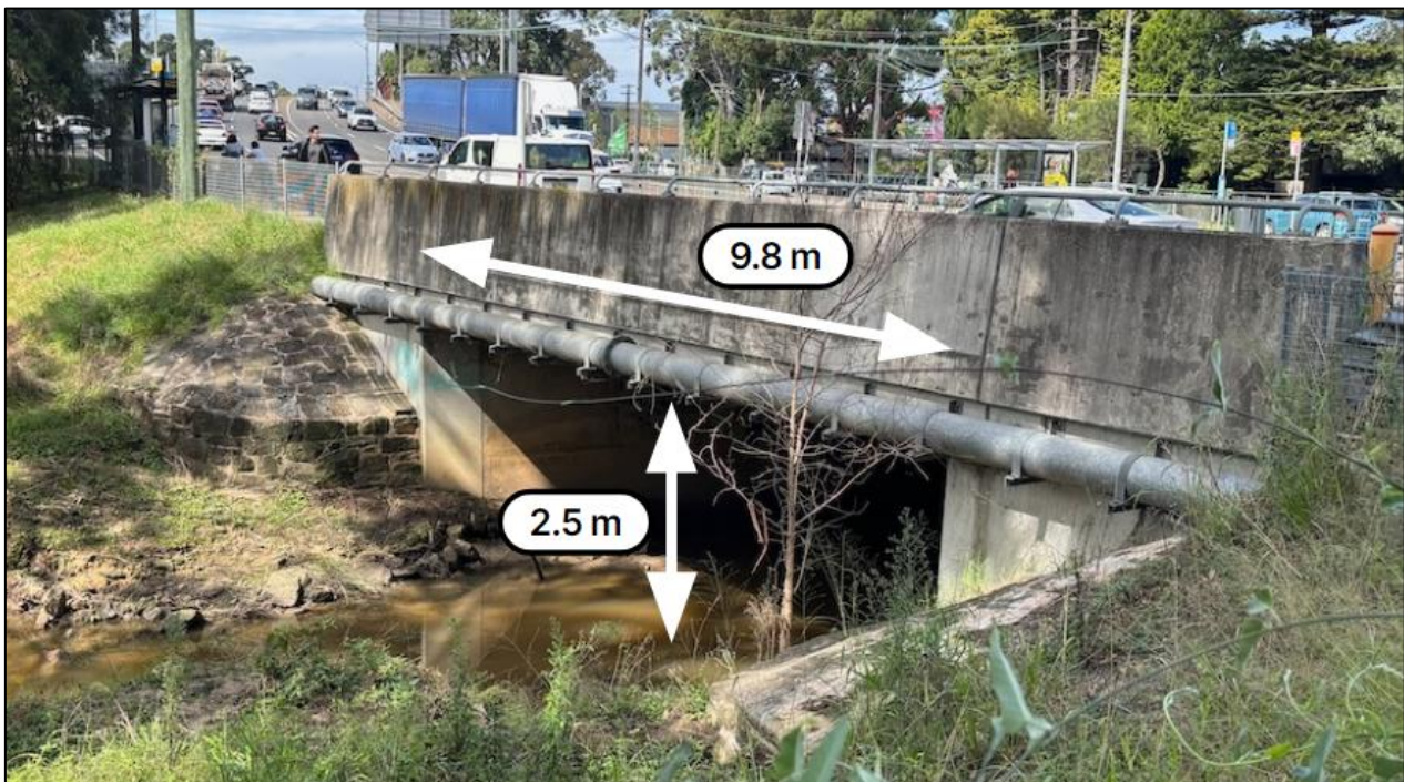
Image 1: Victoria Road Bridge Deck and approximate dimensions (Upstream side)
