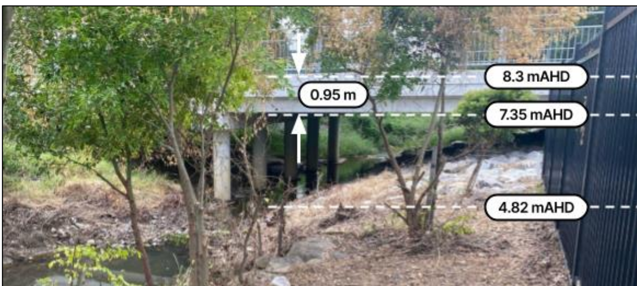
Image 2: Parramatta Light Rail Bridge (Upstream side)
