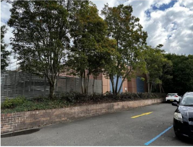
Figure 6 Existing single storey campus central plant building contained to the west of the P1 car park
