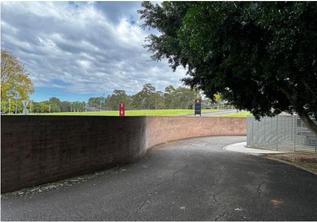
Figure 8 Existing access along western boundary of site to service the single storey plant building
