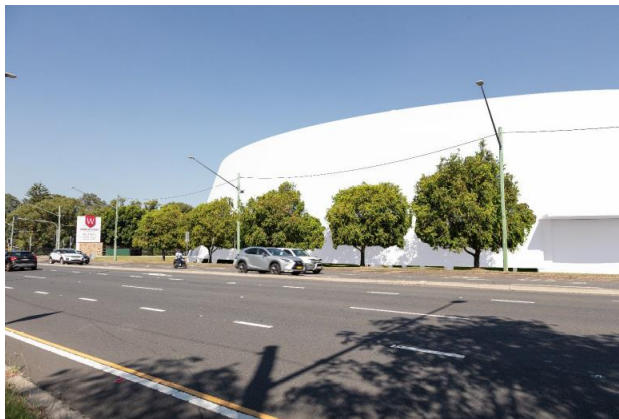
Figure 35 Viewpoint 2 – Victoria Road west: likely future view
