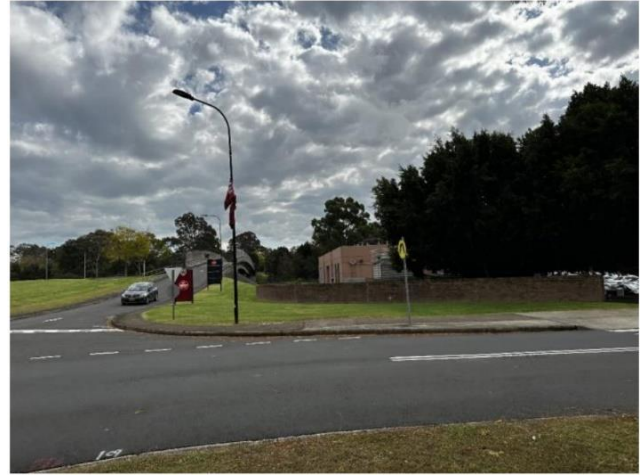
Figure 7 Existing vehicle north-south Victoria Road overpass bridge to the west of the P1 car park
