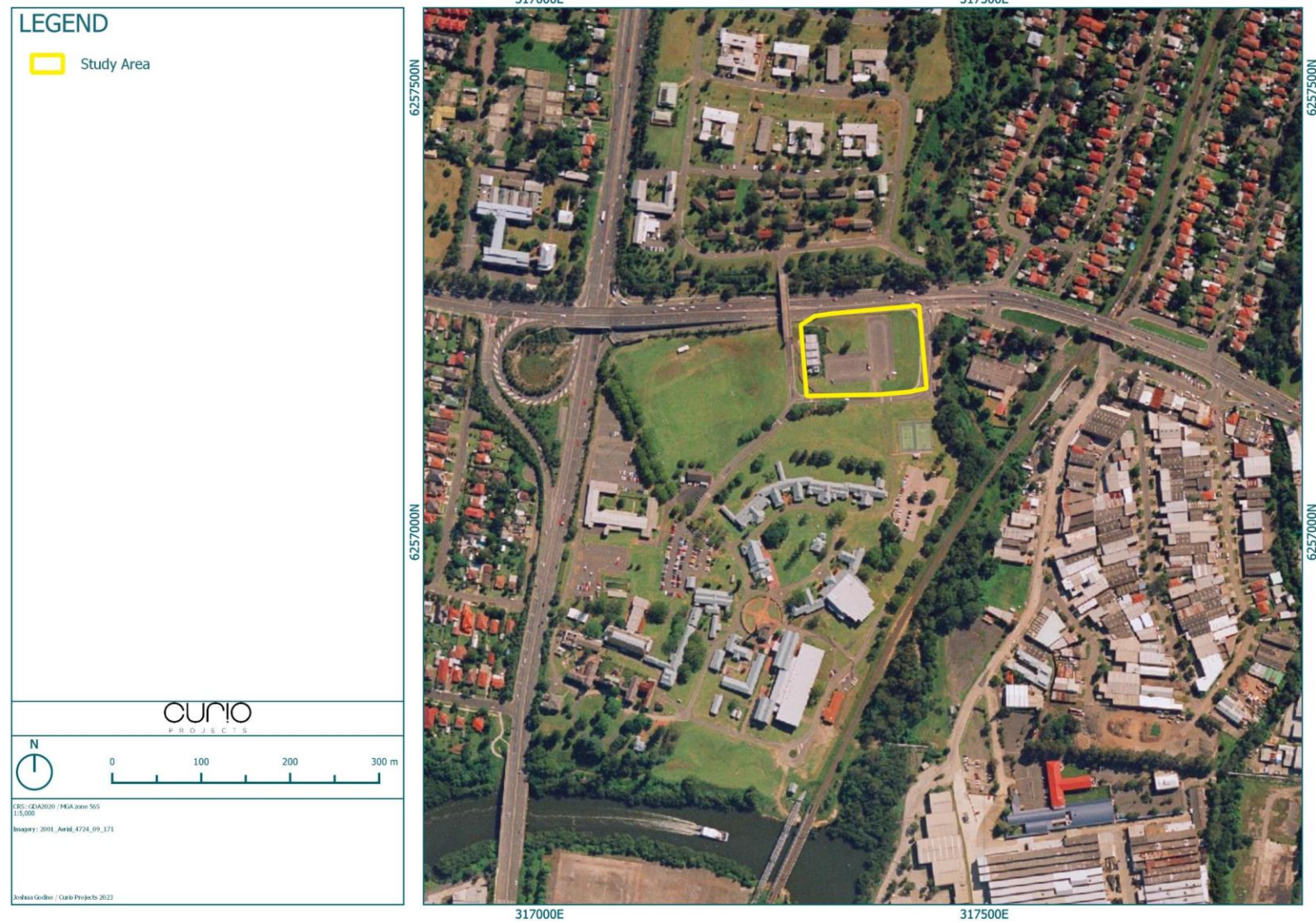
Figure 3-19: 2001 aerial photograph of the study area showing the completed carpark, the Co-Generation Plant Building (Eda) and landscaping. Source. NSW Government SDHI.
